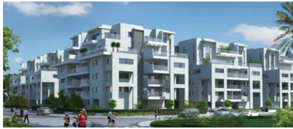
FIG. 5.29 Cramim compound, Shoham, 2013. (Fogel Shoham Architects and Planners) – note that the third floors are larger than the lower ones
