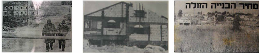
FIG. 3.38 Nirit under construction - Brought in (Pinhas, 1987); (Yediath Ahronot, 1987); (Glick, 1988)
