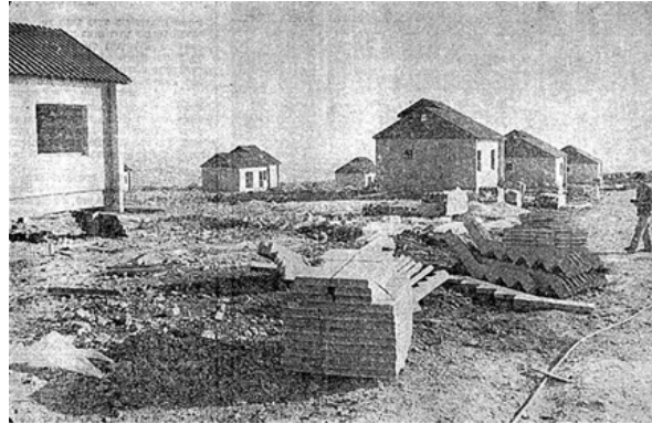
FIG. 3.16 Houses in Reihan during construction, 1980. (Ma'ariv Newspaper)
