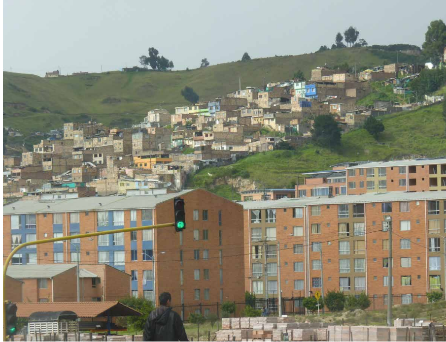
FIGURE 1.1 Mid-rise buildings built in 2010-2012 in Bogota, Colombia. (Photo credit: Rosa E. Donoso)
