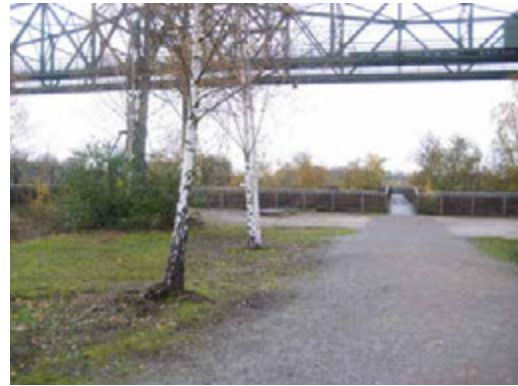
b Bunker roof entrance area. (Photo: Author).
