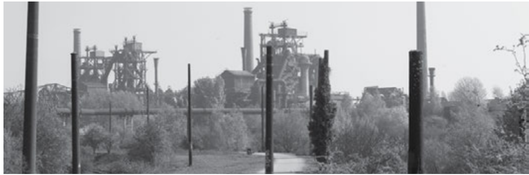
FIGURE 7.60 Rail Harp. (Photo: Dick Sijtsma).
