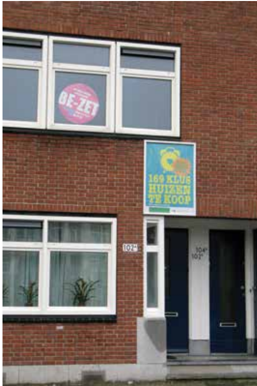
1 Signs of Klushuizen and Be-zet (another housing initiative)
