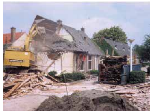
4 Demolition in Tarwebuurt in the early 1980s
