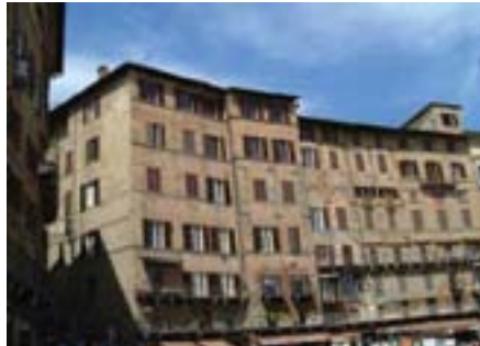
Figure 3.15: Low share of window area at the Piazza del Campo in Siena.
