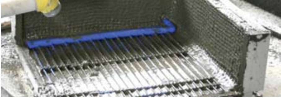
Figure 7.8 Inserting capillary elements into fibre reinforced concrete
