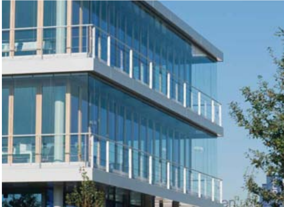
Figure 7.29 Exterior view of the double façade (Solarlux Bissendorf)
