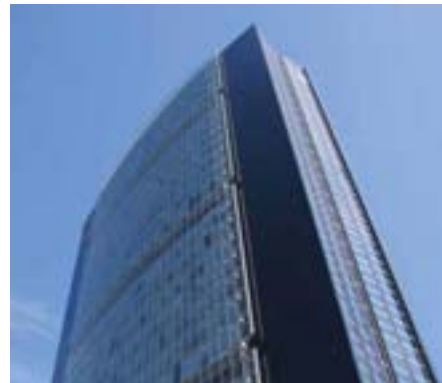
Figure 4.7: ARAG Duesseldorf, Foster and Partner with RKW, 2000 Shaft-box façade: The gap is minimised and designed such that supply air streams in across individual storeys whereas exhaust air is heated in a shaft within the façade and thus rises upward.
