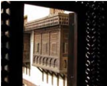
Figure 3.20: By providing shading, the Mashrabiya oriel offers sun protection and good ventilation.
