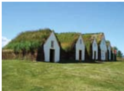
Figure 3.4: Earth covered houses in Island (Michael Scaduto)
