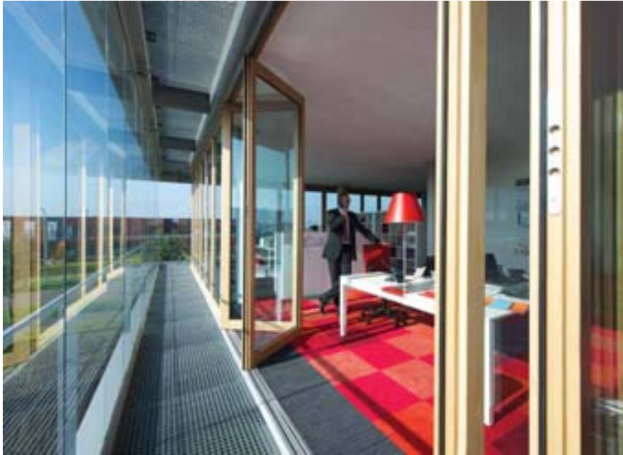
Figure 7.31 View into the double façade space (Solarlux Bissendorf)
