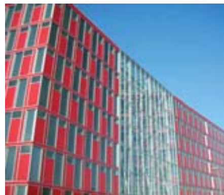
Figure 4.9: Capricon Duesseldorf, Gatermann und Schossig 2006 Component façade with modularised building services components as well as an integration of daylight directing and artificial light facilities.
