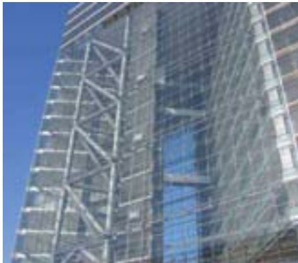
Figure 4.6: Stadttor Duesseldorf, Petzinka, Pink und Partner, 1998 Corridor façade: The outer pane (function: tightness and solar penetration) and the inner façade (function: wind tightness and room enclosure) are almost one metre apart.
