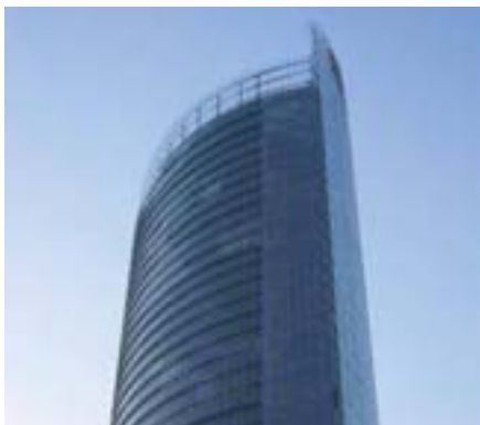
Figure 4.8: Post Tower Bonn, Helmuth Jahn, 2003 Component façade with integration of decentralised heating and cooling devices in a double façade.
