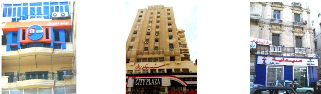
Fig.2: Trespassing material criteria by using materials, not consistent with the old building. Reference: Photographed by the author.
