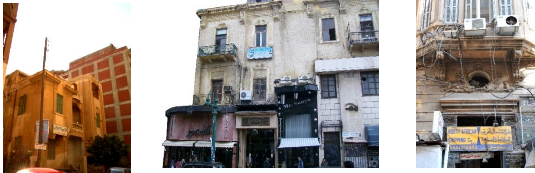
Fig.1: Trespassing structure criteria by heights, commercial use and electrical wires. Reference: Photographed by the author.
