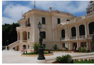
Fig.14: Corridor facade after the adaptive reuse.
