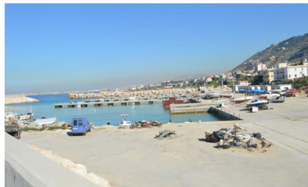
Fig.13: Al-Qalamoun Pier. Source: Researcher
