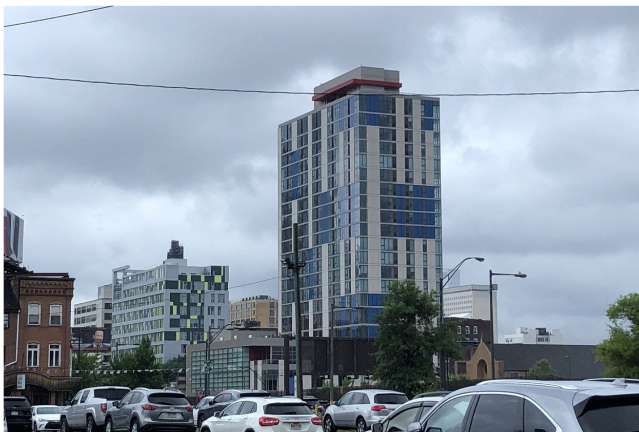
View of the Eastern Tower looking north. Via Philadelphia Inquirer
