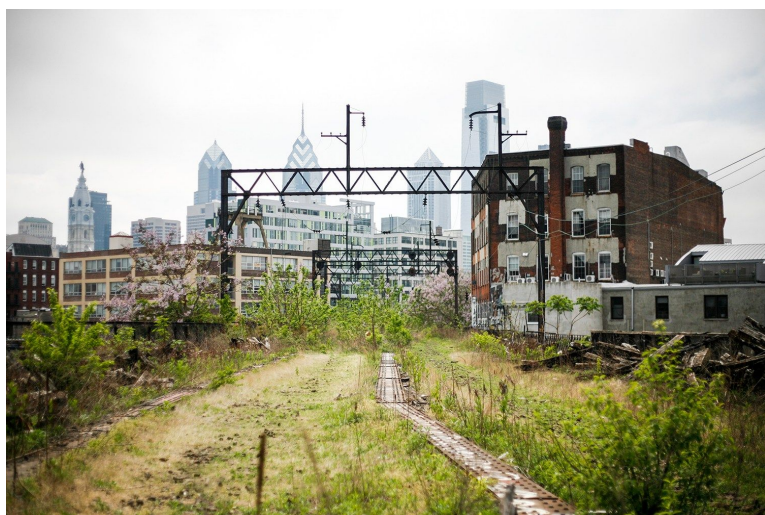
Abandoned trestle pre-Rail Park via Reading Viaduct Project website
