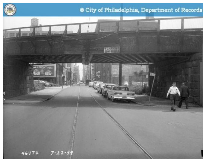
View of trestle pre-Rail Park in 1959, from 12th St. looking south. Via PhillyHistory.com
