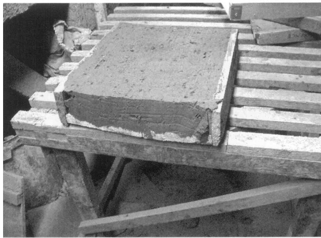
Plate 2.42: Surface left after wiring
