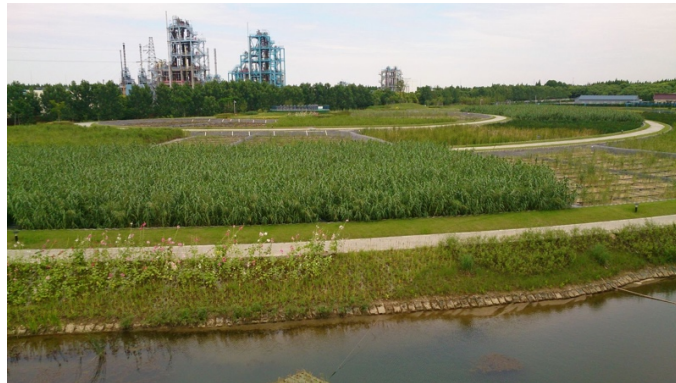
Figure 6. VSSF Constructed Wetland (Blumberg Engineers 2015).
