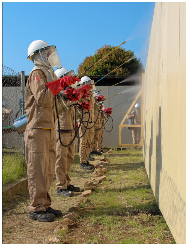
Fig. 1. Mobile wall units used for the training of spray operators in southern Mozambique.
