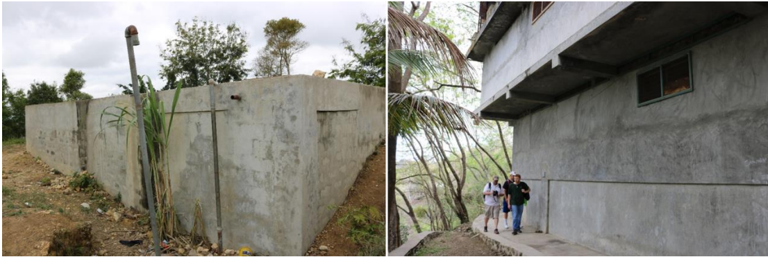
Figure 11. Two water storage cisterns. The one on the left was constructed partially underground and the one on the right is located under a hospital dormitory on the Zanmi Lasante compound.
