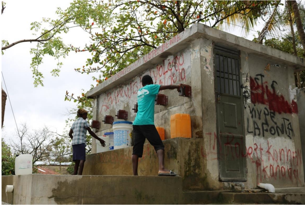
Figure 12. An example of one of the eight fountains located throughout Cange. The fountains have several spigots where water can be collected as well as showers in the rear.
