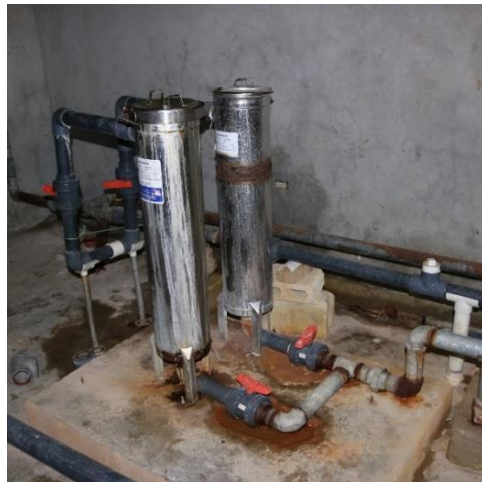
Figure 18. In-line chlorinator made from old system components
