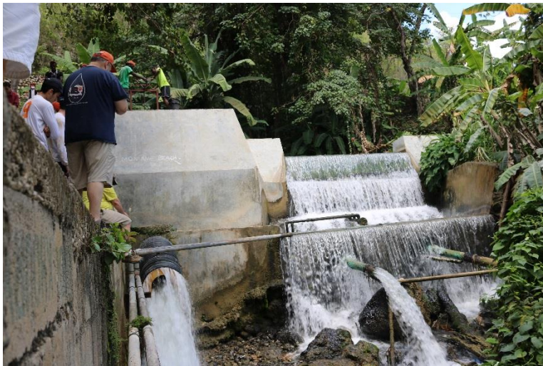
Figure 8. Dam commissioned in 2012 that allowed for system expansion.
