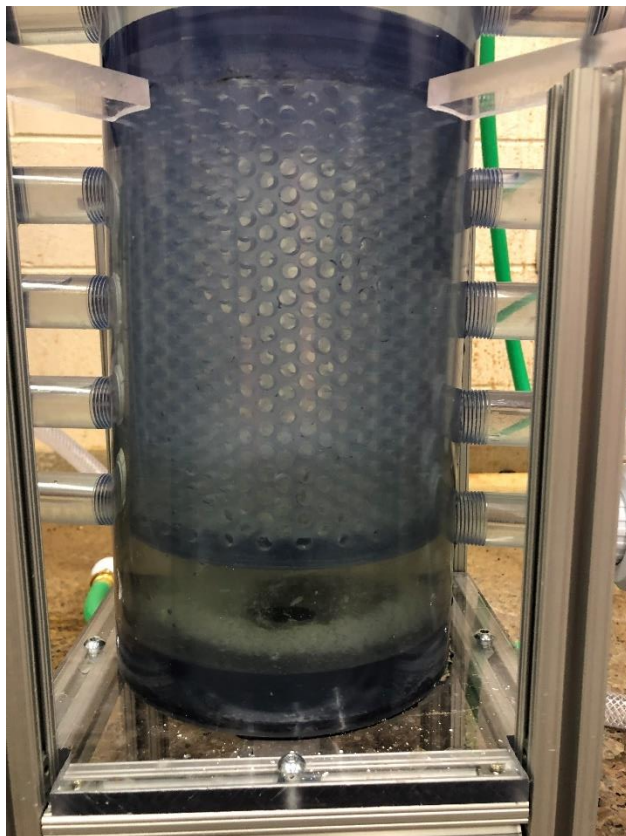
Figure 67. Flakes of the tablet accumulating at the bottom of the chlorinator.
