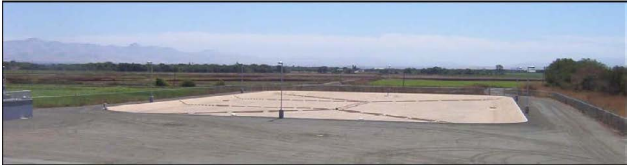
Figure 4. Photograph of Final Constructed Reservoir
