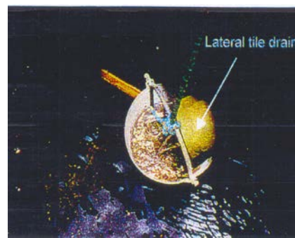
Figure 7. Discharge Measurement in inspection chamber
