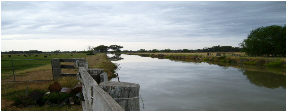
Photo 1. Typical earthen irrigation supply channel
