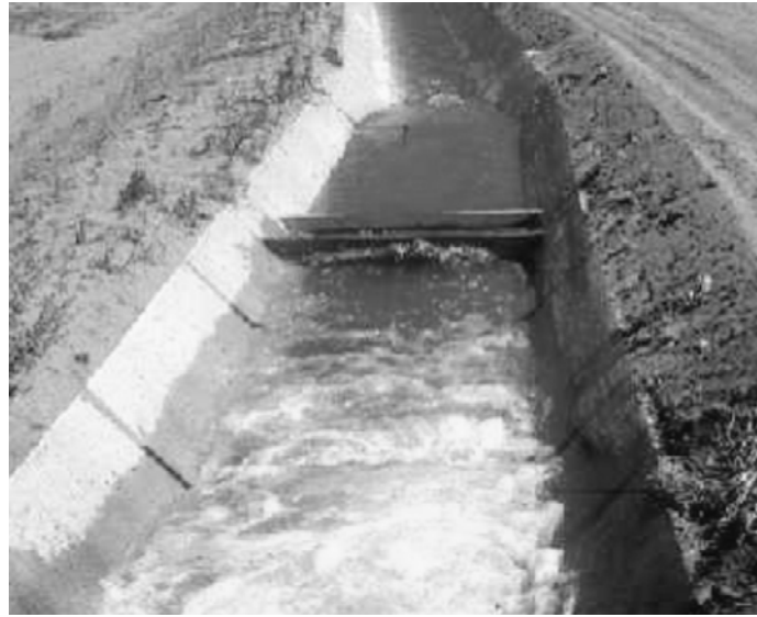
Figure 6. Wave Suppression in Small Canal.
