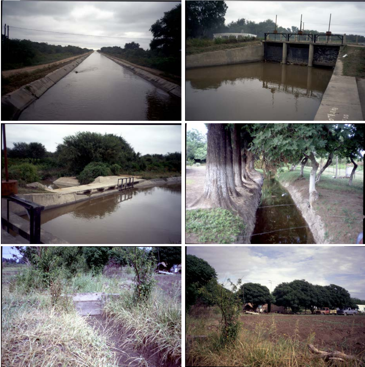
Upper left: San Martin downstream of first cross regulator Middle left: emergency spill upstream of first cross regulator Lower left: farm intake from field canal to field
