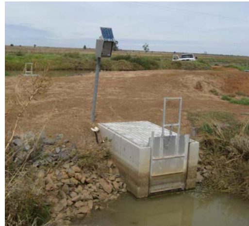
Figure 9. Tyco Irriflow EM Meter – Transducer (left) and Turnout Installation (right)
