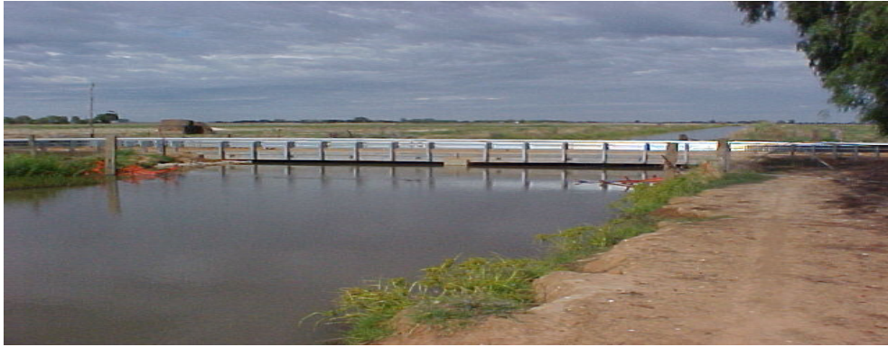
Photo 2. Typical earthen irrigation supply channel
