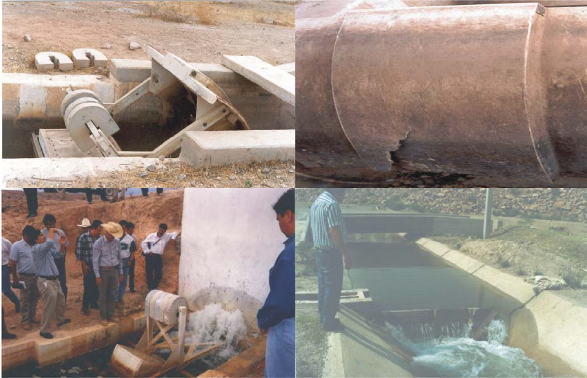
Figure 2. Damage and hydraulic instability of Self-Leveling Gates
