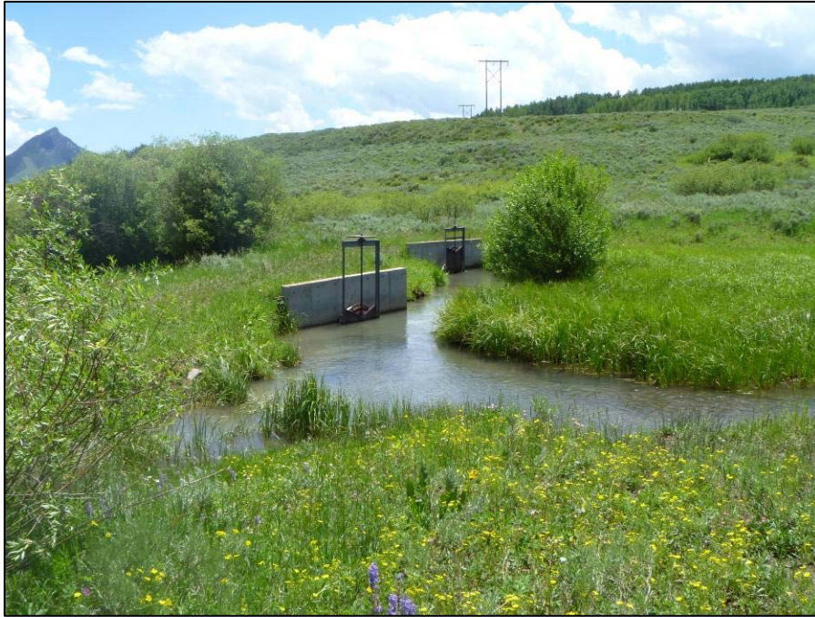
(C). Diversion of Little Muddy Creek at Martin No. 1 Ditch. Example includes two headgates; one in middle foreground blocks downstream flow to creek, one in middle background releases flow into ditch.
