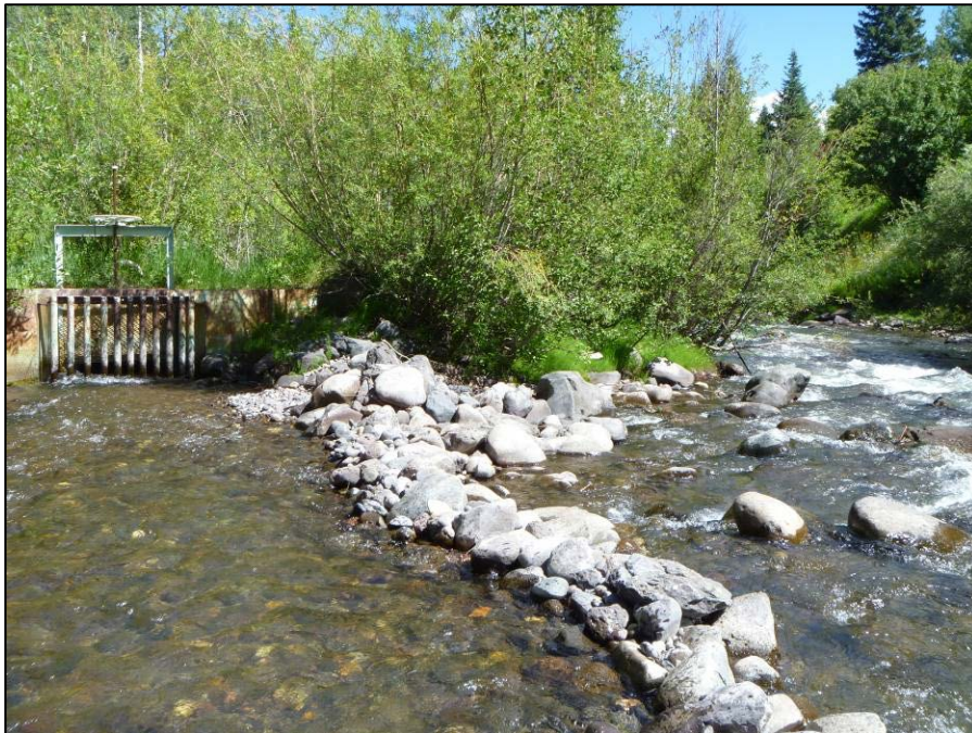
(D). Diversion of East Fork Williams Fork at Egry Mesa Ditch. Example of a rock weir with metal headgate. Williams Fork was not surveyed in this study, due to flows exceeding those safe for wading at the potential control reach site.
