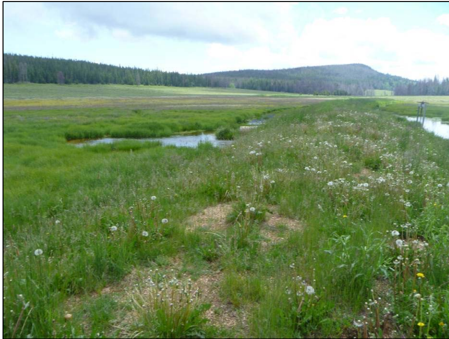
Figure 8. Examples of diversion and headgate types for study sites. (A). Diversion of Service Creek at Sarvis Ditch headgate. Berm blocks and collects flow from Service Creek and wetland, diverting it into ditch on right side of berm in image.
