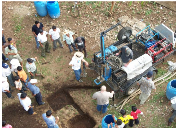
Figure 4.7 Drilling a well in Guatemala
