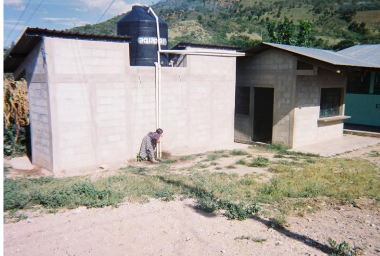
Figure 4.3 Finished water cistern and gravity fed tap at the school in Los Encuentros
