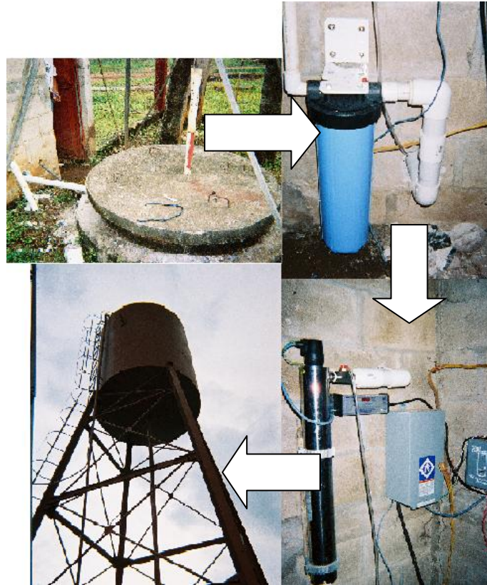
Figure 4.5 The water treatment process for La Nueva Cajola
