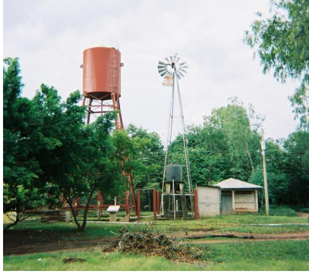
Figure 2.1 Donated Red Cross water tower in Guatemala
