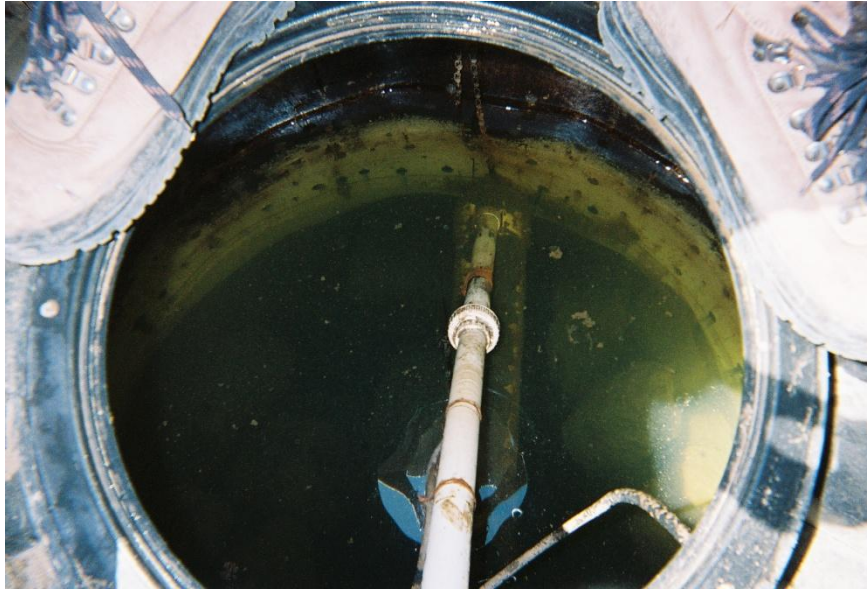
Figure 4.1 Alluvial well in Los Encuentros (note the perforated tank sides)
