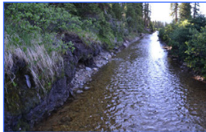
Ditch diverts groundwater flow from fen to reservoir
