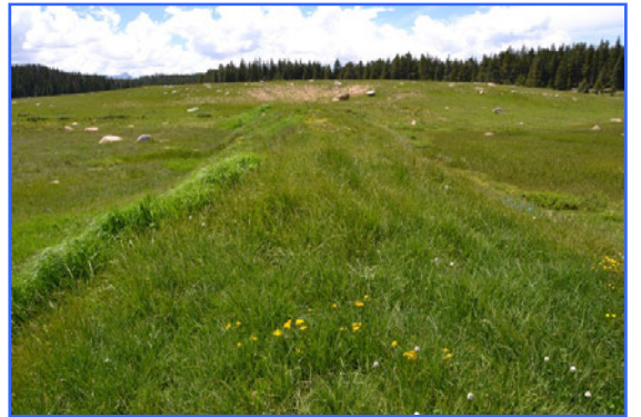
Dam alters groundwater flow to fen
