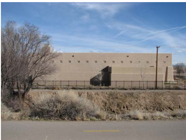
Alameda Pump Station
