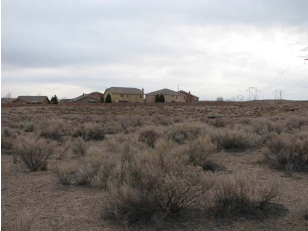
Ladera Dam System Managed by AMAFCA (Adjacent to a residential zone.)
