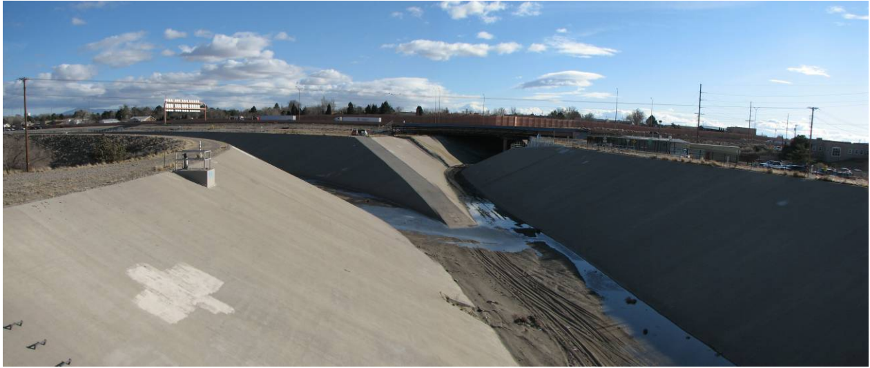
North Diversion Channel (Confluence of Enbudo Channel)
