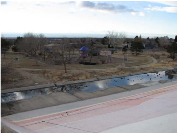
Piedra Lisa Park (The park works as a detention basin.)
