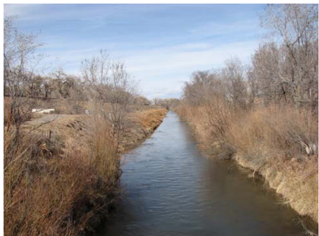
Albuquerque River Side Drain (Managed by MRGCD)
