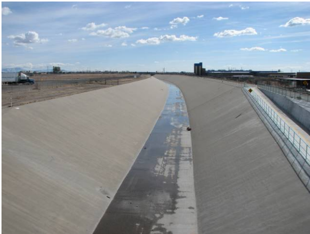
North Diversion Channel (Alameda Blvd)
