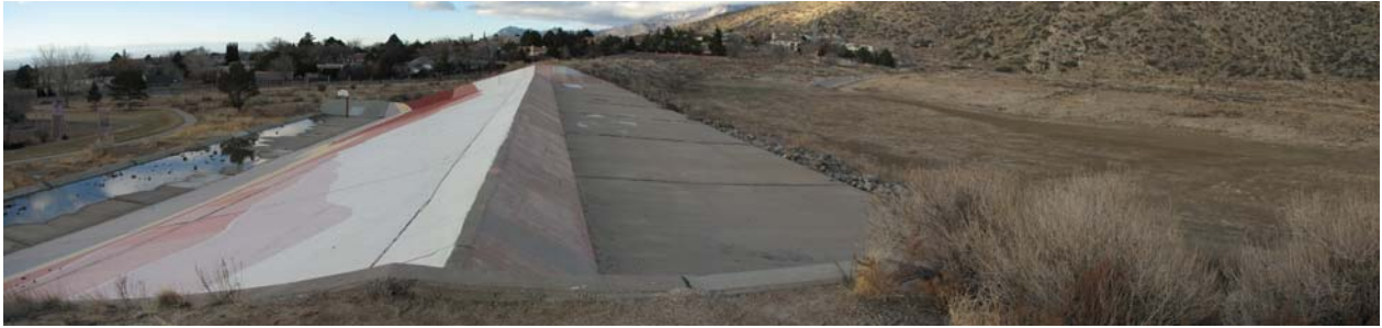
Piedra Lisa Dam (Managed by the City of Albuquerque)
