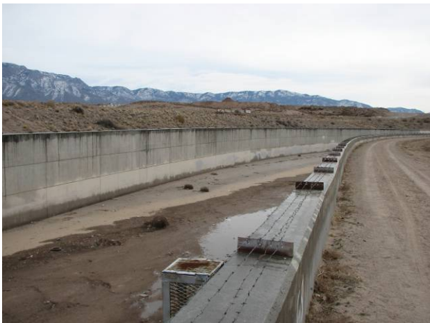
North Diversion Channel (Near Confluence of Rio Grande)
