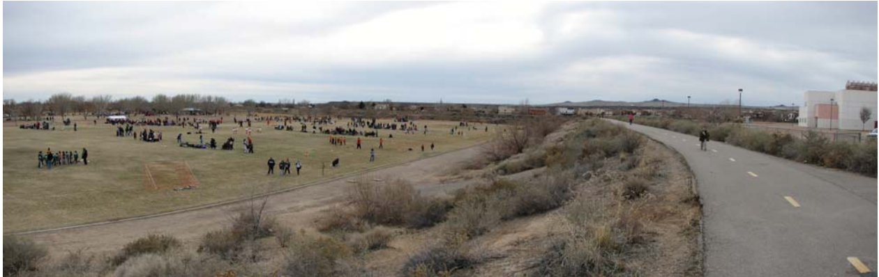
Mariposa Detention Basin Managed by the City of Albuquerque (Utilized as a sports ground.)
