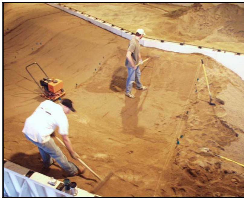
Figure 3.6: Placement of Backfill between Model Sections During Construction
