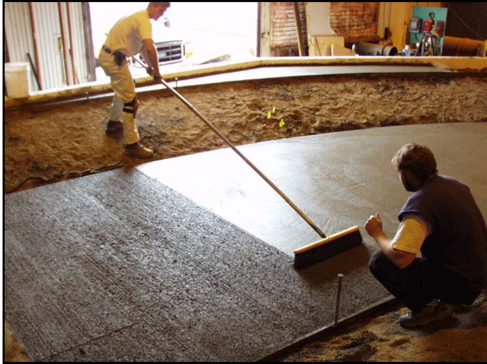
Figure 3.7: Placement and Roughening of the Concrete Cap
