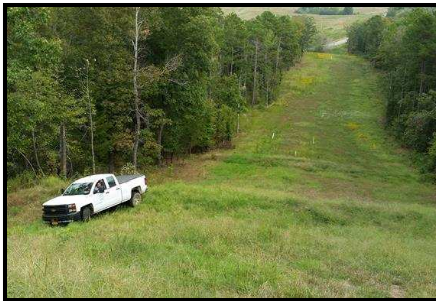
Figure 47 ROW with a steep slope, but mowed and relatively accessible.
