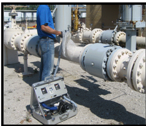
Figure 19 Operator performing a high-flow measurement of a leak emission at TDTS.
