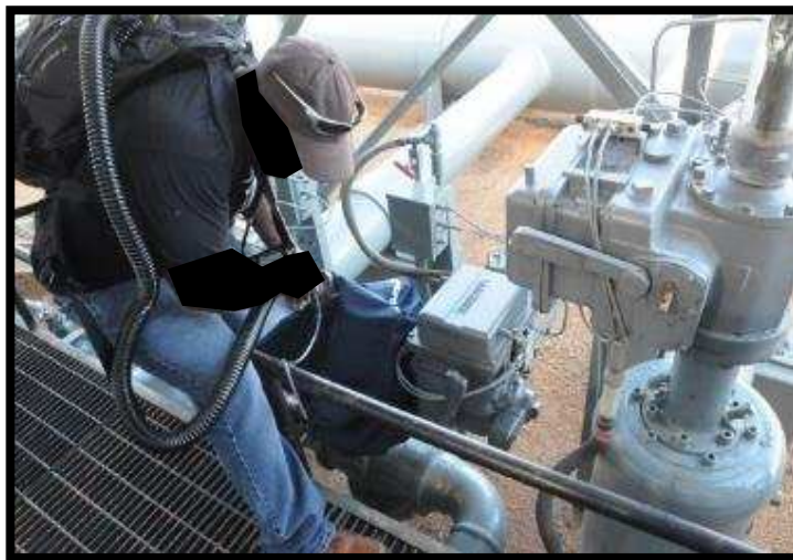
Figure 7 Bacharach high flow setup using an inherently safe enclosure placed over the leaking device to obtain a complete capture of emitted methane. The flow is routed and analyzed in the operator's backpack and then recorded by the operator.
