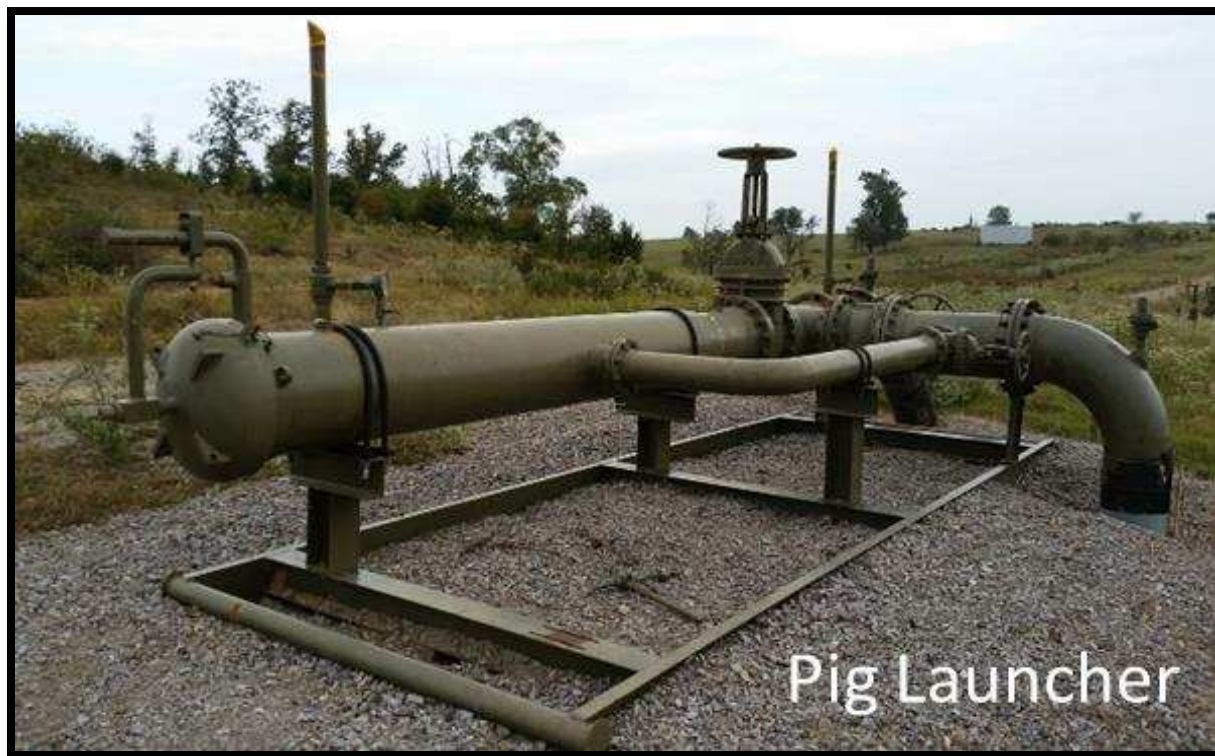
Figure 42 A typical pig launcher/receiver from the study area. Door or hatch to the pig launcher can be seen on the left side of the image.
