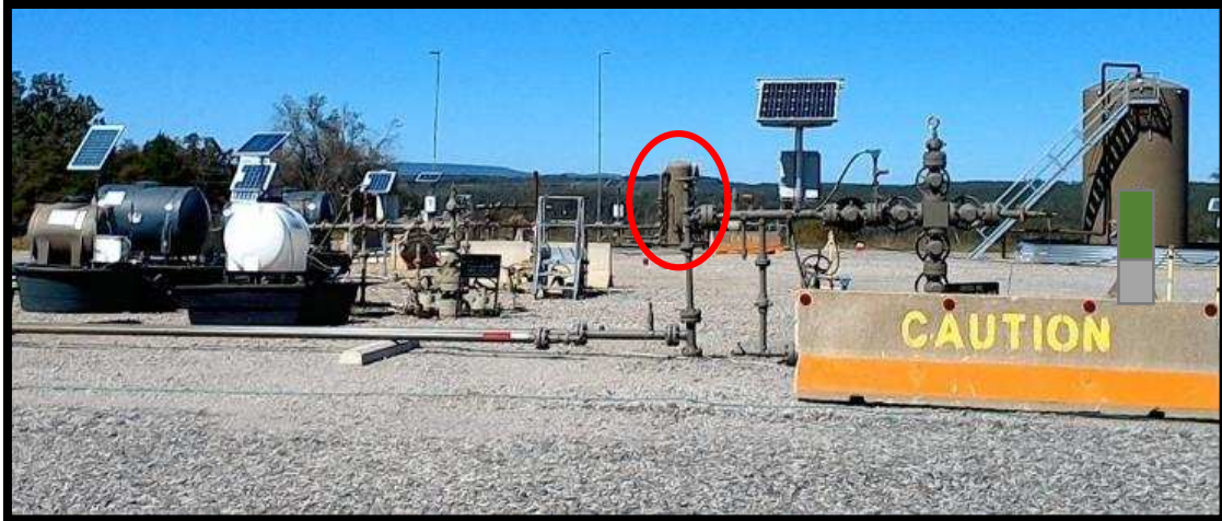
Figure 2 Production well pad, no compressor or plunger present on the well tree to assist in gas lift. Glycol and foamer tanks present at the left of the image, vertical separator highlighted with a red oval. Produced water tank at the right side of the image.
