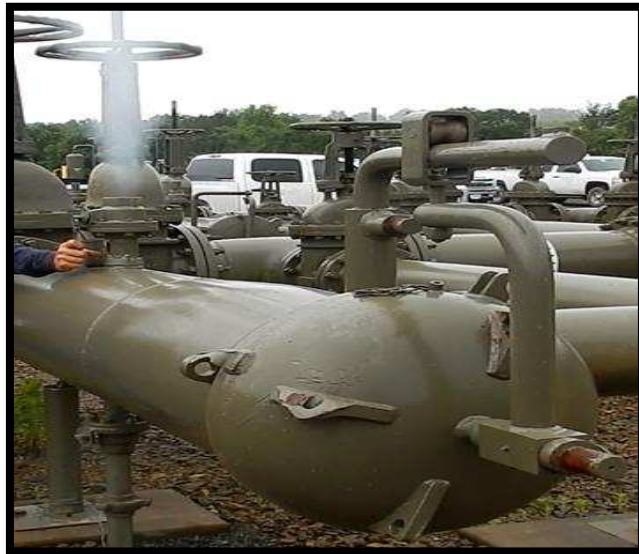
Figure 59 Venting of Pig Launcher Chamber
