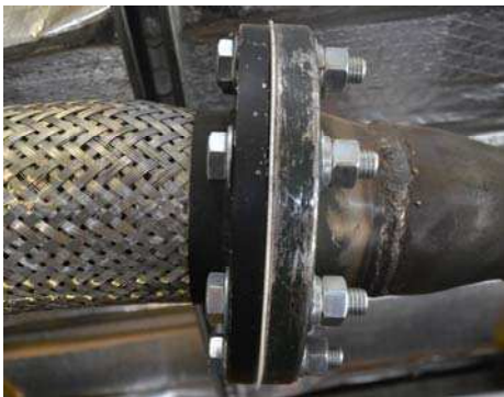
Figure 4-48. Flanged connection.
