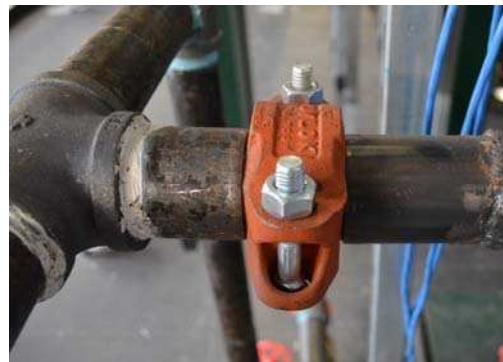
Figure 4-49. Grooved connection.
