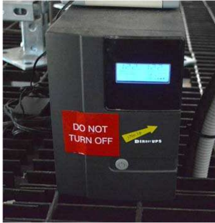
Figure 4-14. The UPS maintains power to EMB systems in a power loss scenario.
