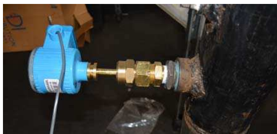
Figure 4-81. Glycol loop insertion style flow meter.
