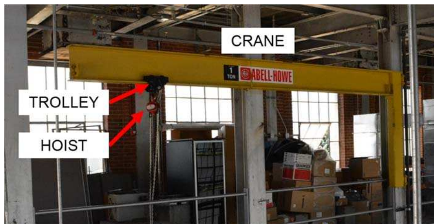
Figure 4-54. Crane installation prior to facility construction.
