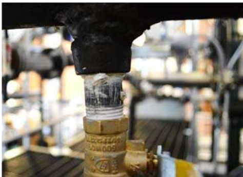
Figure 4-50. Threaded connection.
