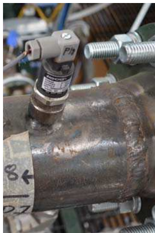
Figure 4-71. Absolute pressure transducer installed in pipe.
