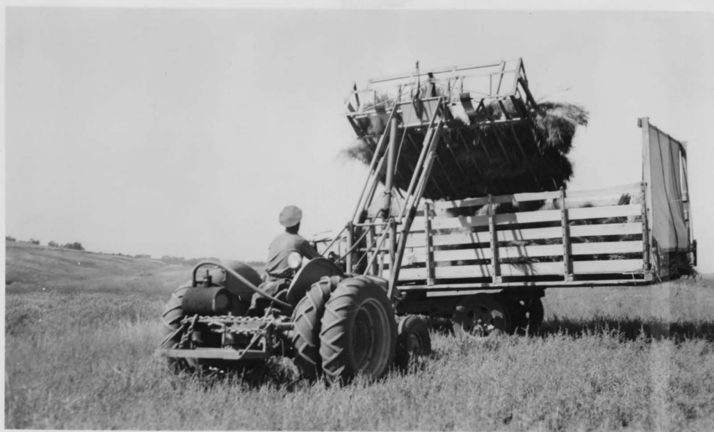
Picture 8.--Loading bundled barley with hydraulic "farm-hand"
