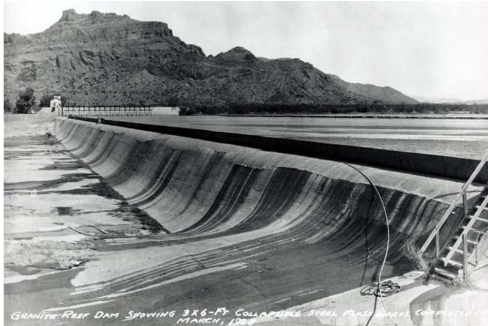
Image 2. Granite Reef Diversion Dam.
