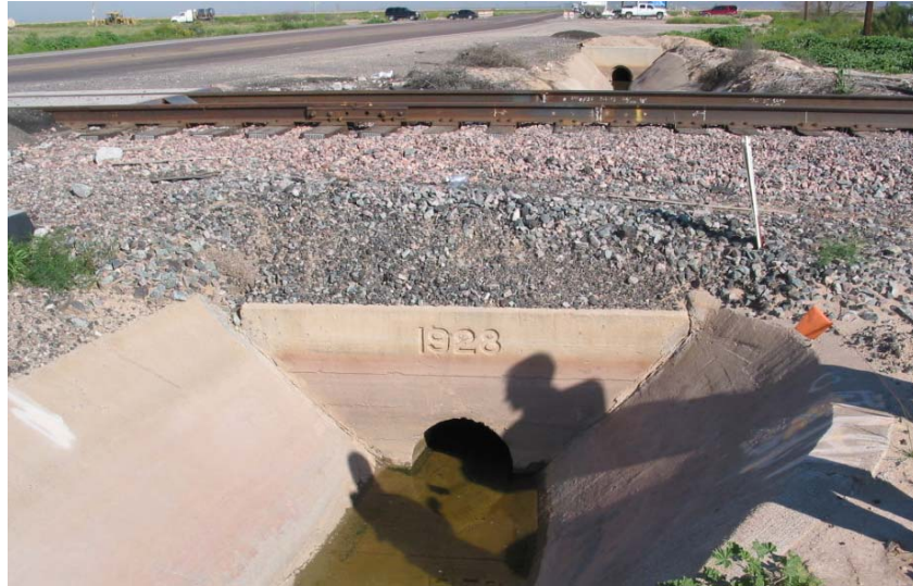
Figure 6. Existing Headwall Constructed in 1928
