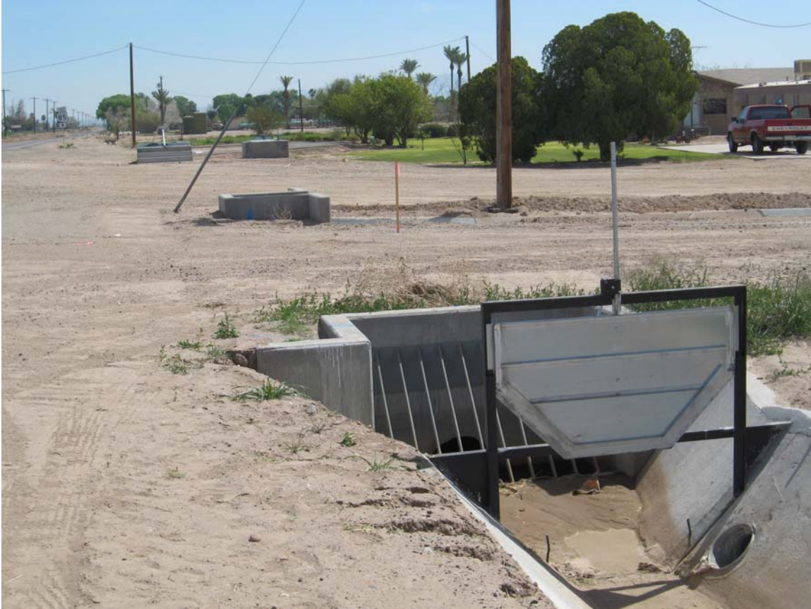
Figure 3. BWCDD Structures and Private Ditch and Gate
