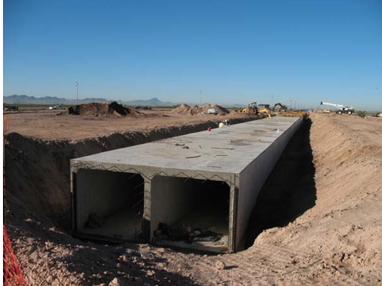
Figure 11. Construction of RID Box Culvert
