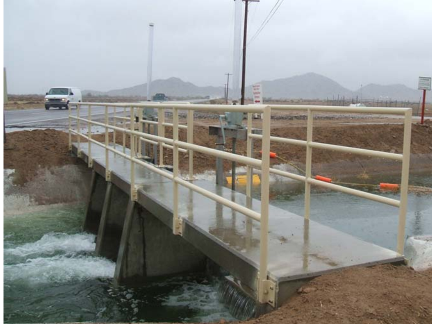
Figure 8. New RID Check Structure
