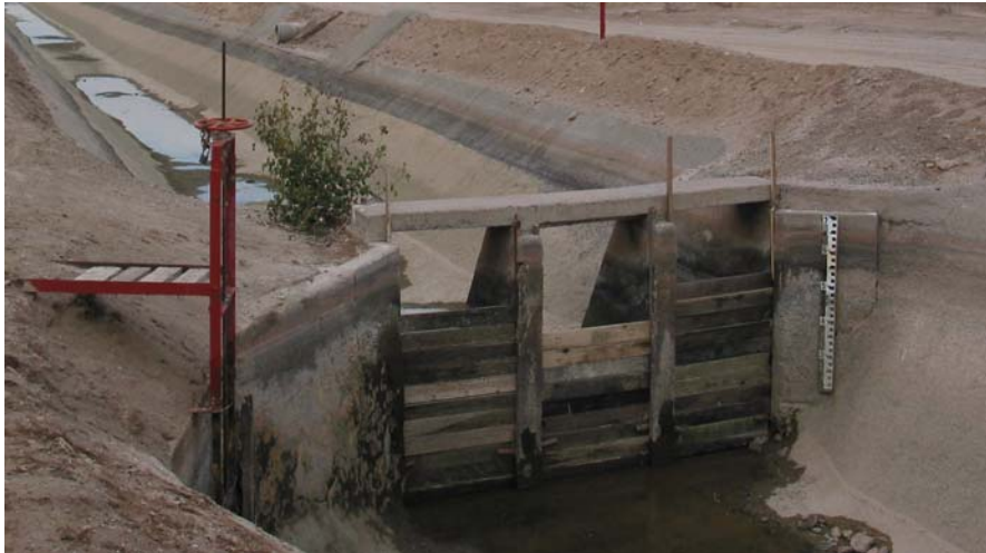
Figure 7. Original RID Check Structure
