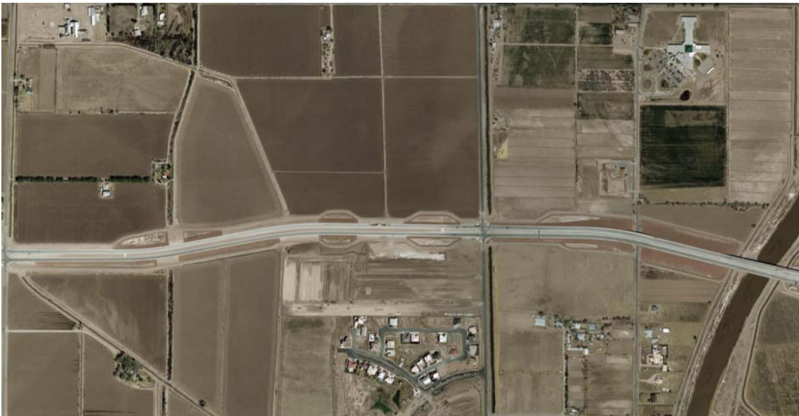
Figure 3. Aerial Photograph of Highway Crossing District Facilities
