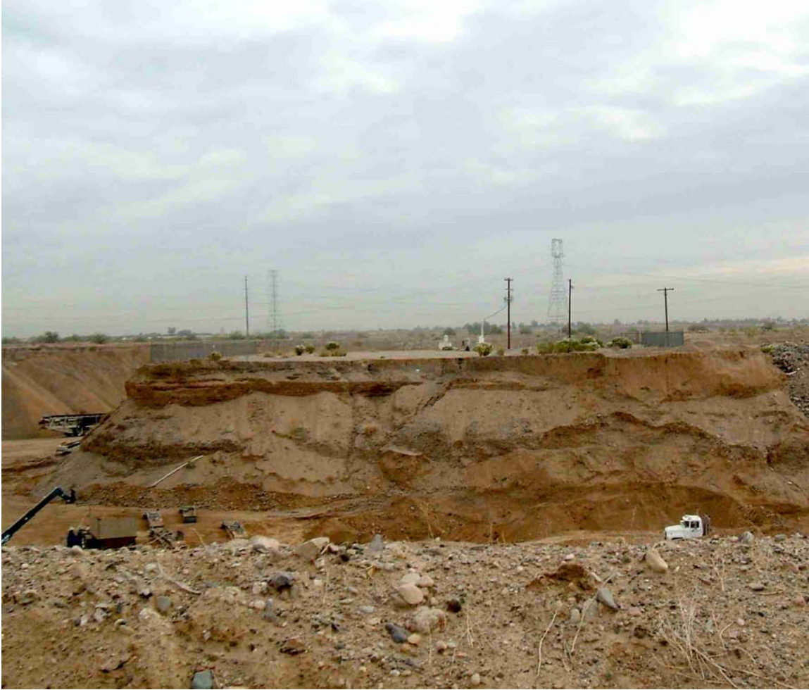
Figure 3. Vertical Mining along Well Perimeter and Loss of Perimeter Fencing
