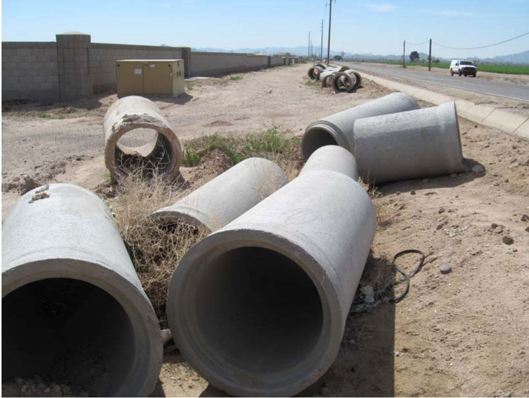
Figure 4. Abandoned pipe waiting to be installed.
