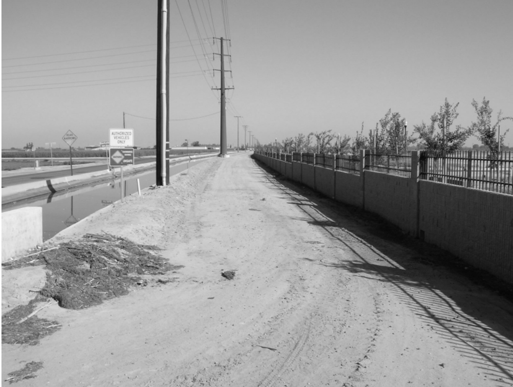
Figure 3. Masonry Wall along Canal
