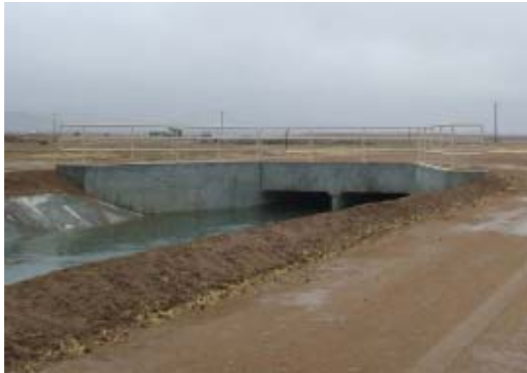
Figure 12. RID Main Canal Final Product
