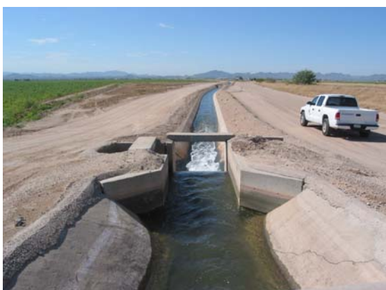
Figure 3. Open Lateral Turnout
