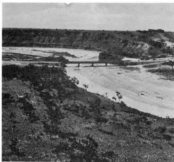
View of the Río Caris gaging site looking upstream. The A35 recorder is attached to the bridge abutment and is visible in the photograph. The river is destroying the riprapped abutment where the recorder is located.
