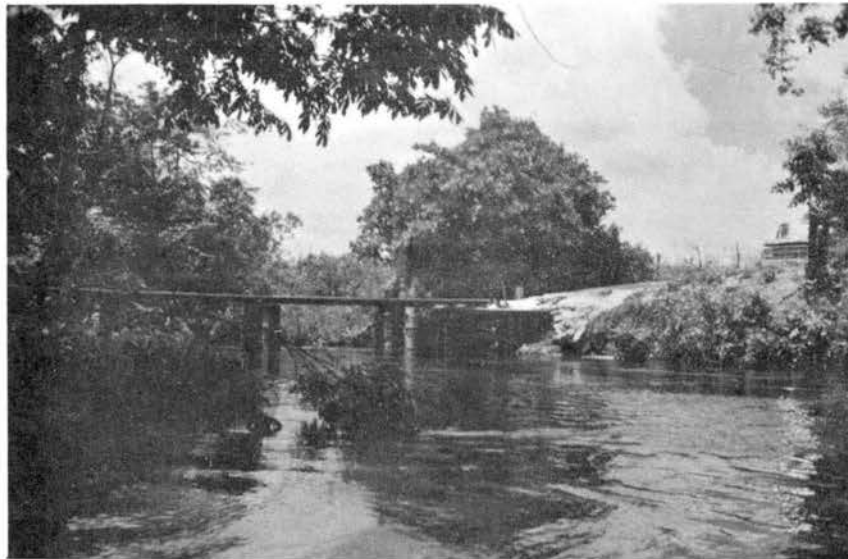
Looking downstream at Río Arco gaging site. The A35 recorder is in the metal house on top of the corrugated metal pipe attached near the right abutment of the bridge. Most of the discharge measurements were made at a section about 100 feet downstream of the bridge.
