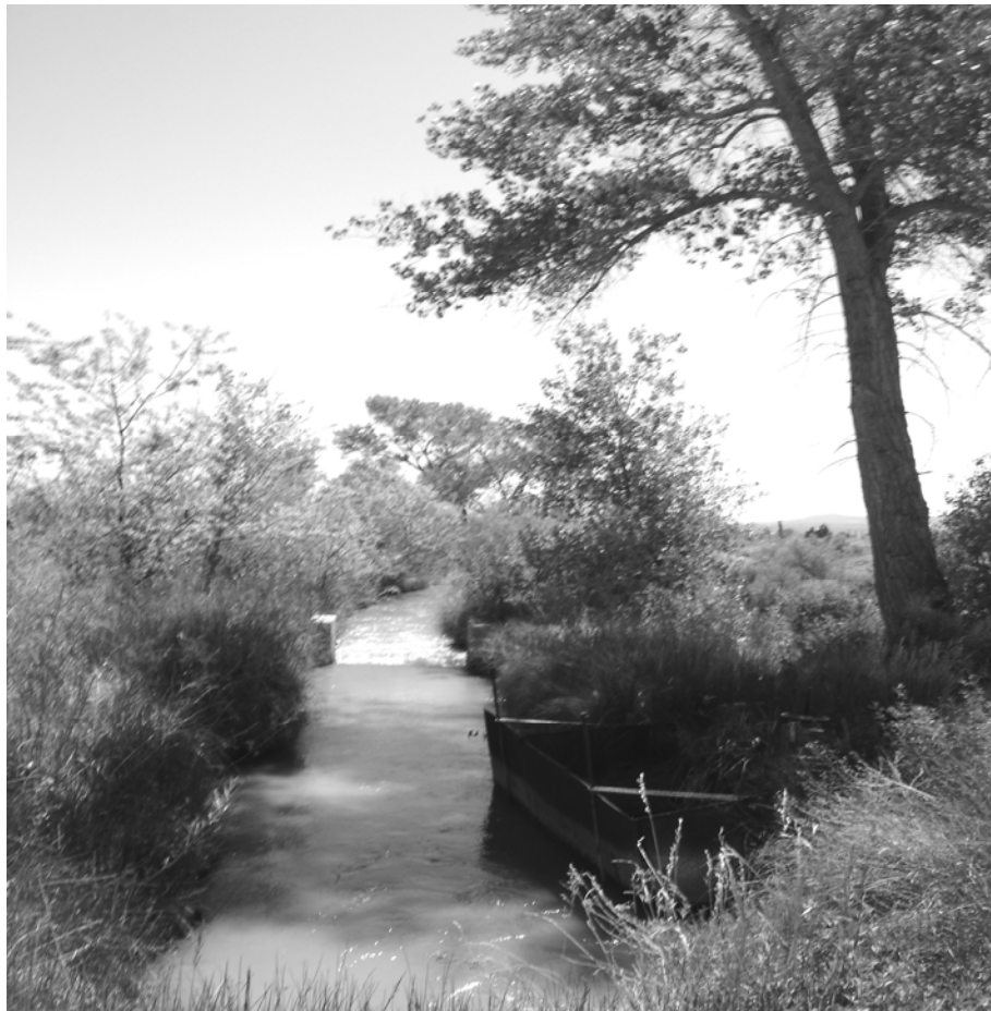
Figure 1. The Huntington-Cleveland Irrigation Company's Cleveland Canal provides an example of wildlife habitat expected to be lost when the canal is replaced with a pipeline.
