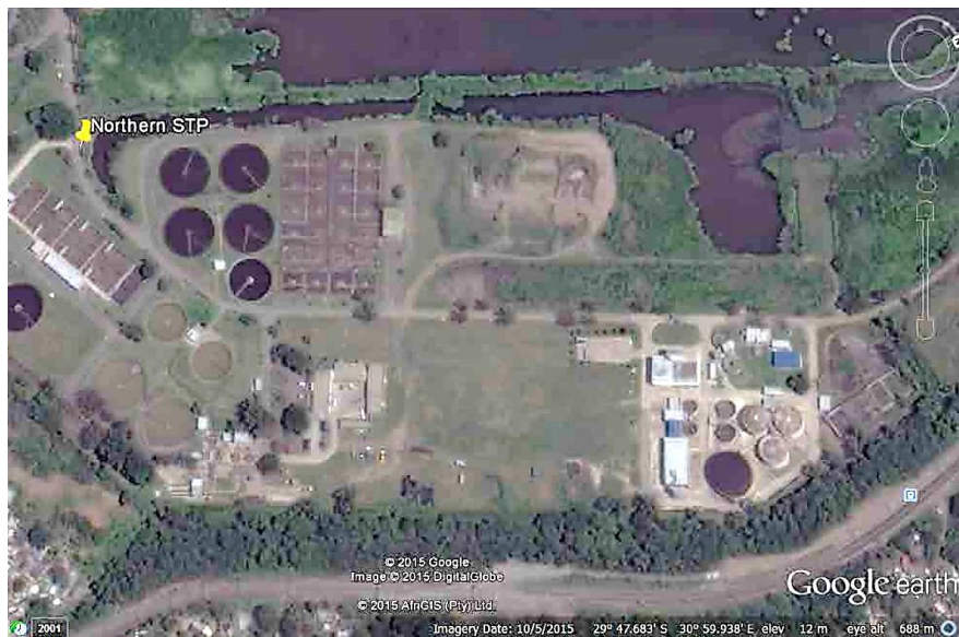
Figure 4.14: Aerial view of Northern Treatment Works. Source: Google Earth, 2015.
