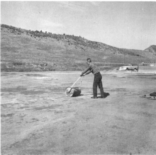
Fig. 25. Repairs were completed by hand rolling
