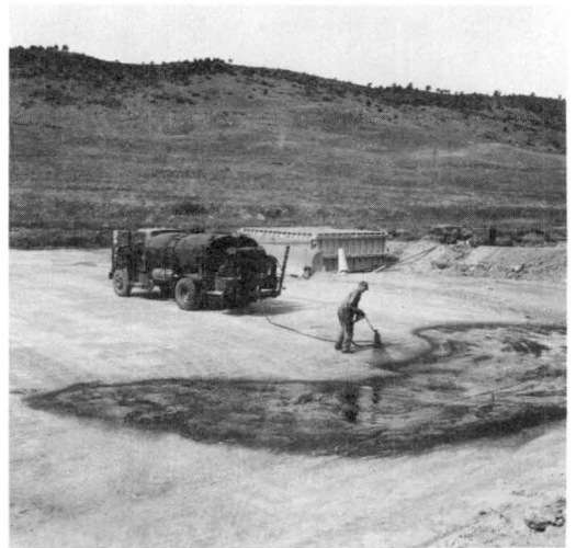
Fig. 10. Prime coat asphalt was used to stabilize the terrain
