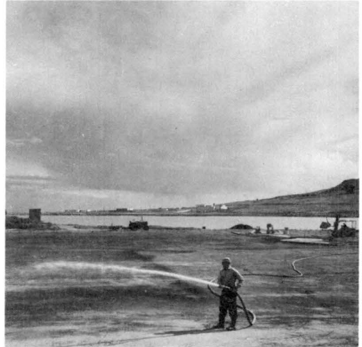
Fig. 8. Sprinkling maintained the proper soil moisture for good compaction.
