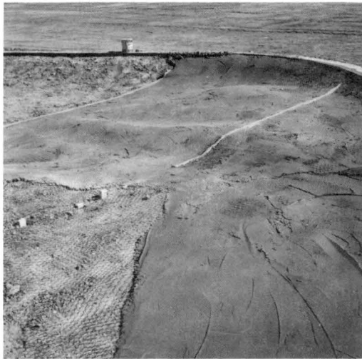
Fig. 17. Wire netting was used as reinforcing for the first coat of concrete
