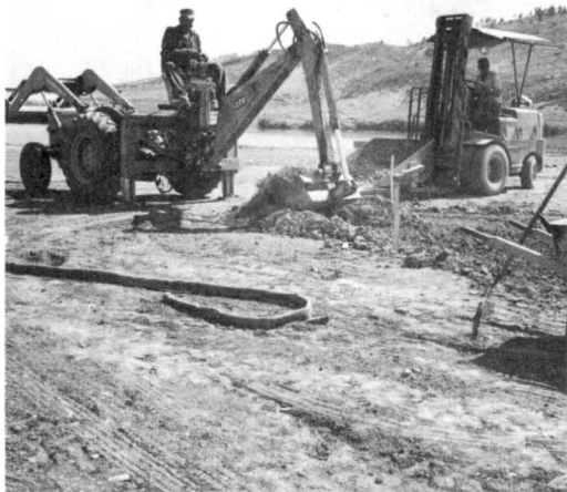
Fig. 3. A tractor mounted backhoe completed the rough topography layout
