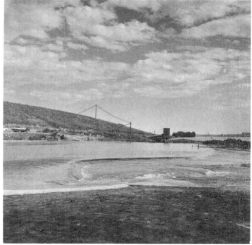
Fig. 20. The crest of the dam became a control at the higher discharges
