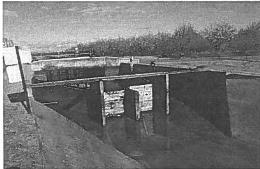
Figure 4 - Long Crested Weir
