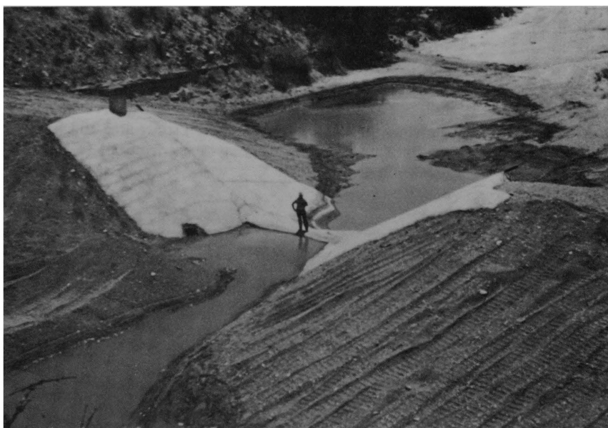
FIGURE 8.—Critical flow flume originally installed for flow measurement at the Walnut Gulch Watershed outlet, 1954. BN-48652
