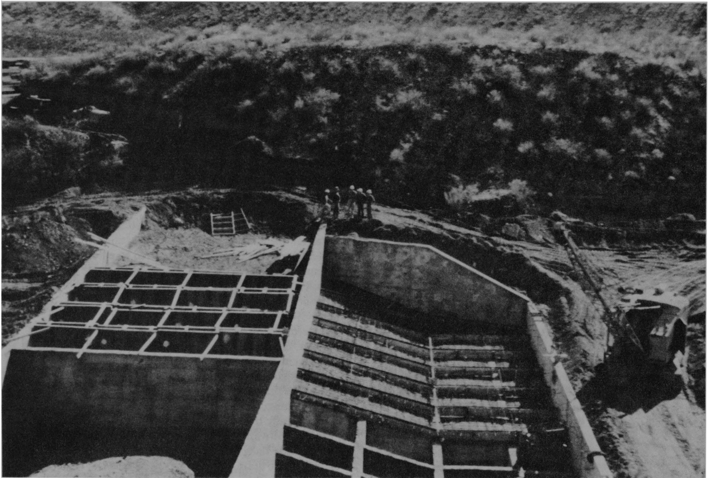
FIGURE 41.—Flume construction in early stages with form construction just beginning. BN-48664
