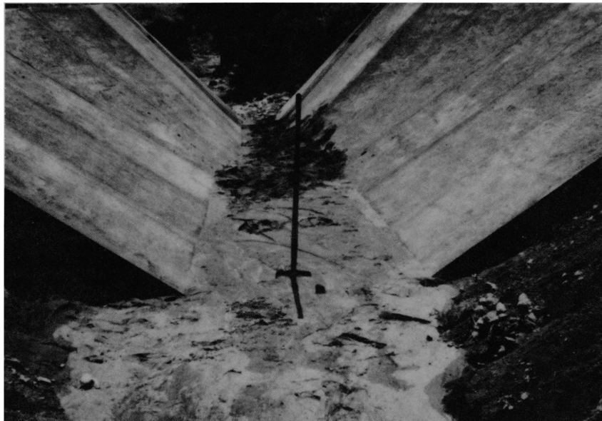
FIGURE 4.—Measured rating of an alluvial filled 2:1 V-notch weir, Walnut Gulch Location 63.102. Only at depths greater than 0.4 to 0.6 m (1.5 to 2 feet) does the weir exert control.
