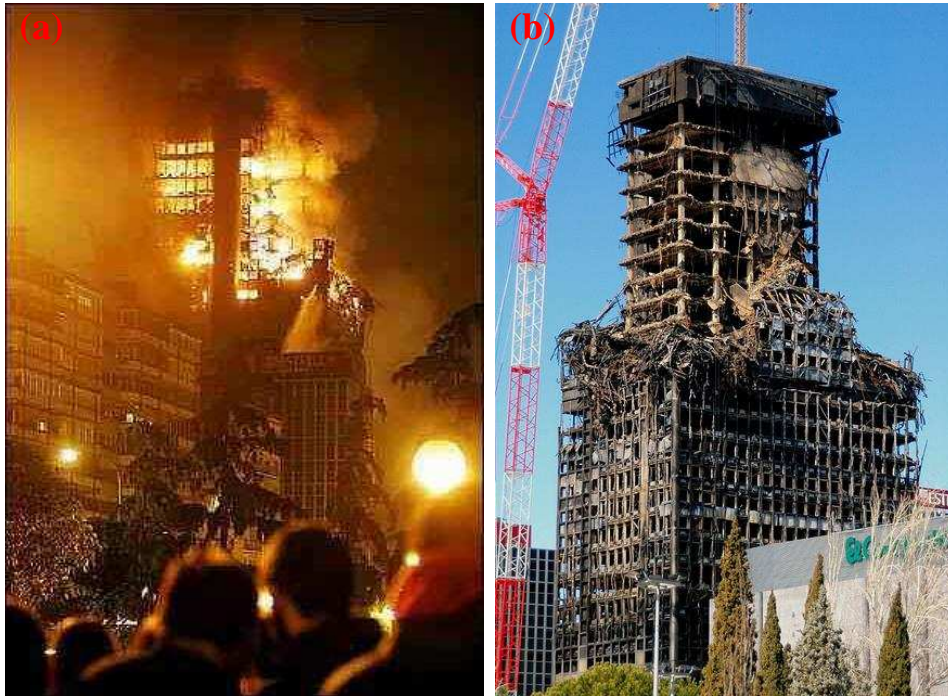
Figure 2.8 (a) Fire flames engulf top 10 stories of Windsor building in Madrid, Spain (b) partial collapse in top 10 stories.
