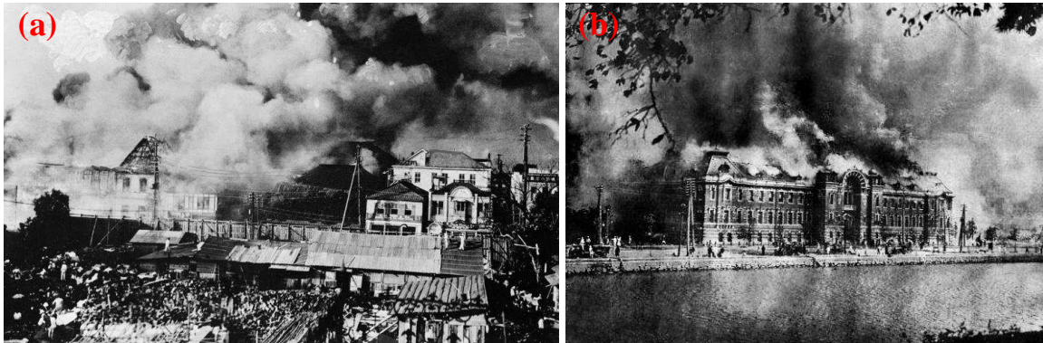
Figure 2.3 (a) Ginza district of Tokyo engulfed in flames after the 1923 Tokyo earthquake (b) burning of metropolitan police department at Marunouchi following the 1923 Tokyo earthquake, photographers unknown.
