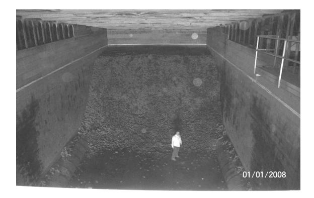
Figure 3. Example of typical bulk storage pile (5 m. pile height) in the San Luis Valley of Colorado
