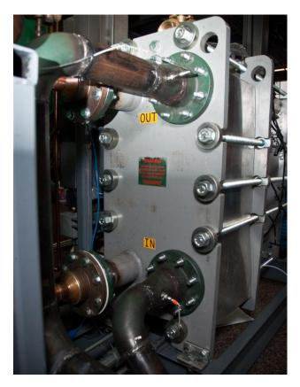
Figure 5-2: Vaporizer as installed with piping.
