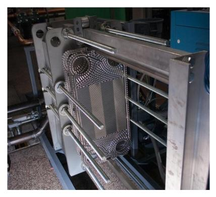
Figure 5-1: Vaporizer with spare individual plates not installed.
