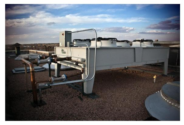
Figure 5-7: Condenser as installed on third floor roof at the EECL.
