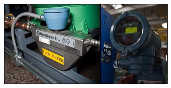
Figure 5-10: Micro Motion coriolis flow meter sensor (left) and transmitter (right).
