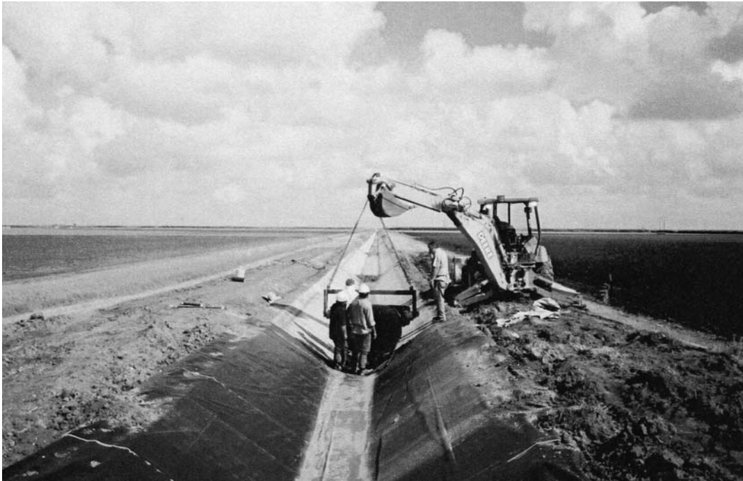
Photo 3. Placement of EPDM Panels by the Irrigation District
