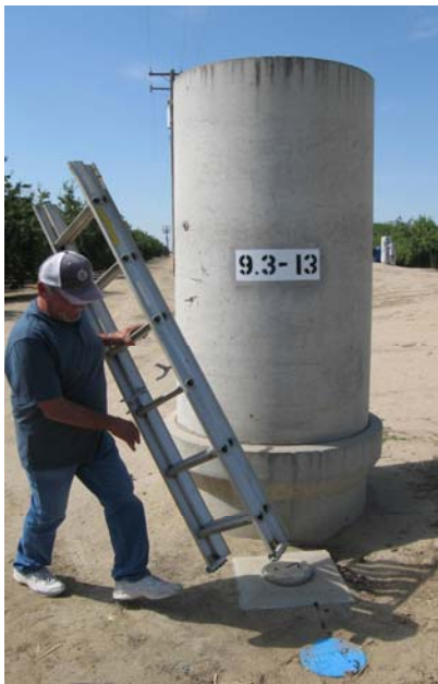
Figure 2. Existing Farm Turnout Standpipe
