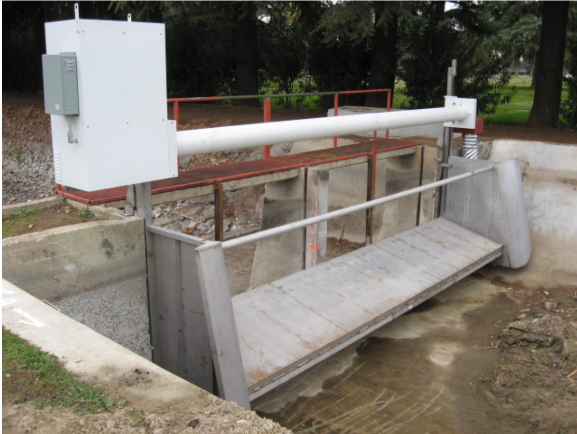
Figure 5. Langemann Gate Used to Automate Headgate
