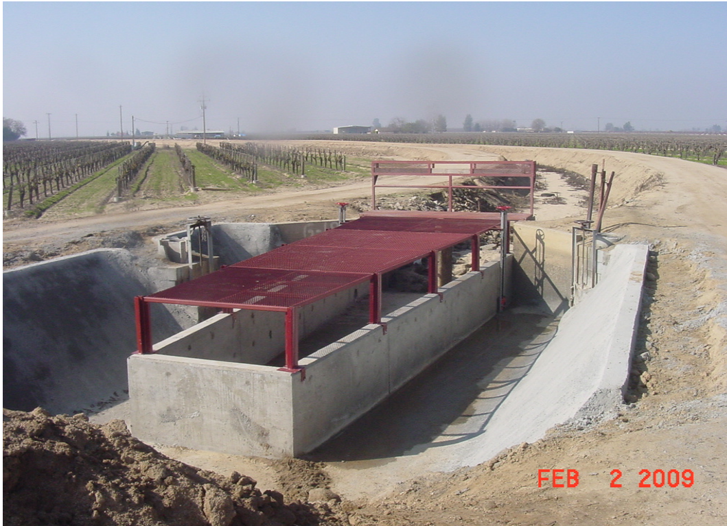
Figure 4. Weir Retrofitted with LCW
