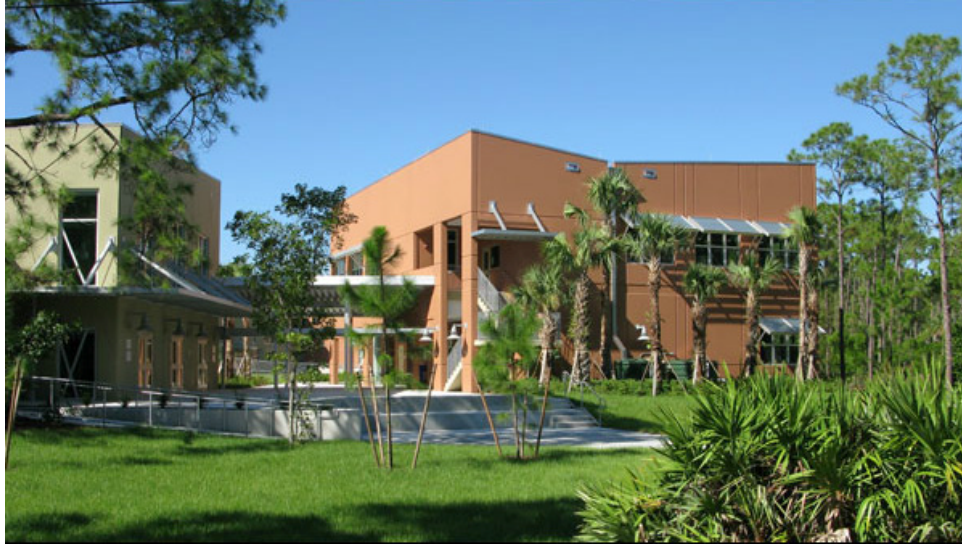
Figure 5. Pine Jog Elementary School 4
