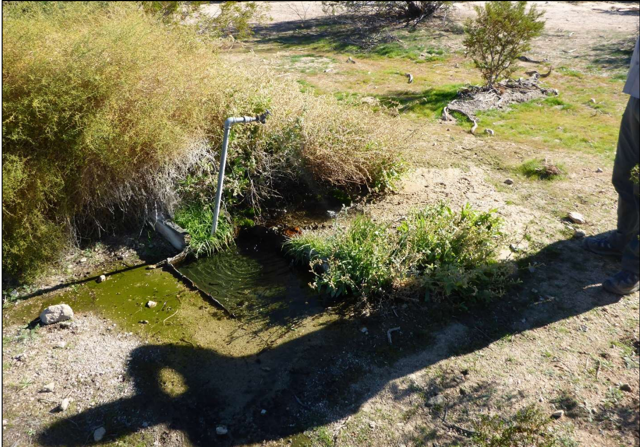
Figure 9-21. The leaking spigot near the generator house, a continual small pool of water is present year-round.
