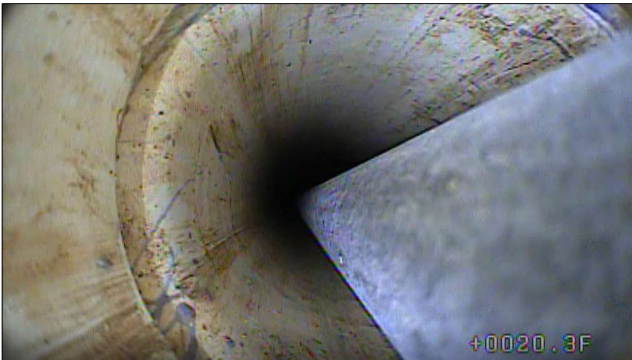
Figure 9-15. Camera screenshot inside LUB-23 at a spool length of 20.3 ft, and 17.9 ft below ground surface (the well entry point is 2.4 ft above ground surface). 11/28/18.
