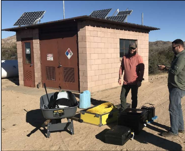
Figure 9-1. Photo of the Generator House. Tyler Gilkerson (left) and John Boyle (right); prior to setup 11/26/18.
