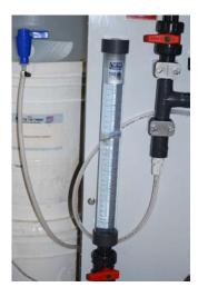
Figure 6 - Pump Calibration Column
