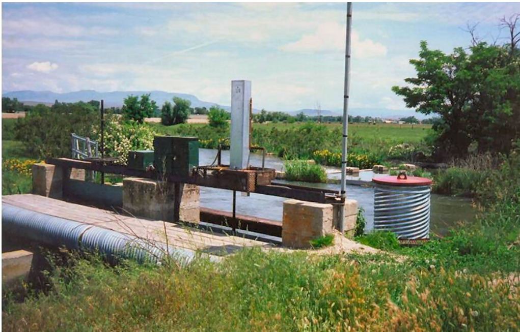
Figure 5. Noble Ditch headworks structure
