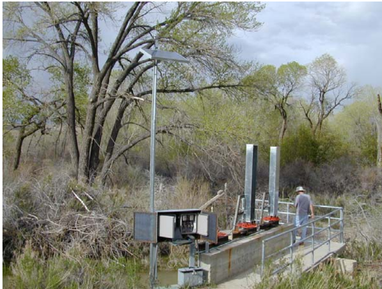
Photograph 2. Gate Actuators Being Installed on Huntington Canal Diversion Structure
