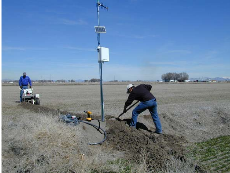
Photograph 5. Installing Soil-Moisture Monitoring Units near Delta, UT
