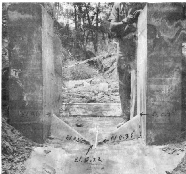
A. Upstream view showing low-water constriction
