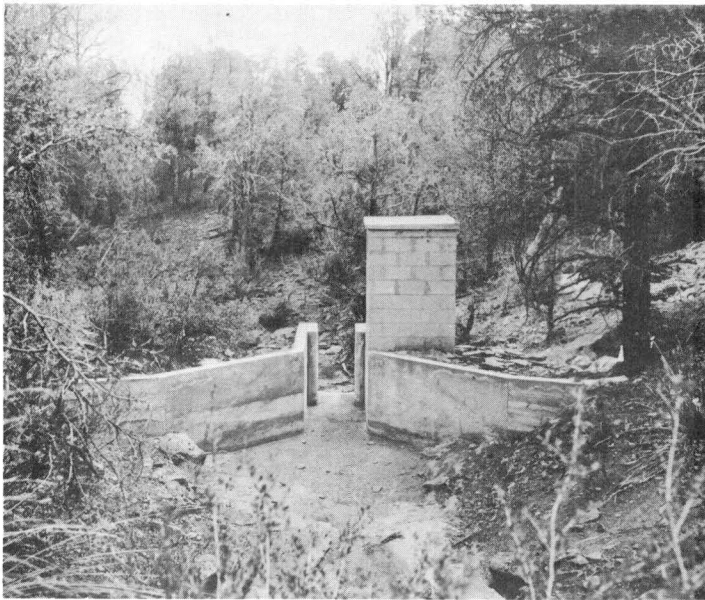
A. Downstream view of gaging station
