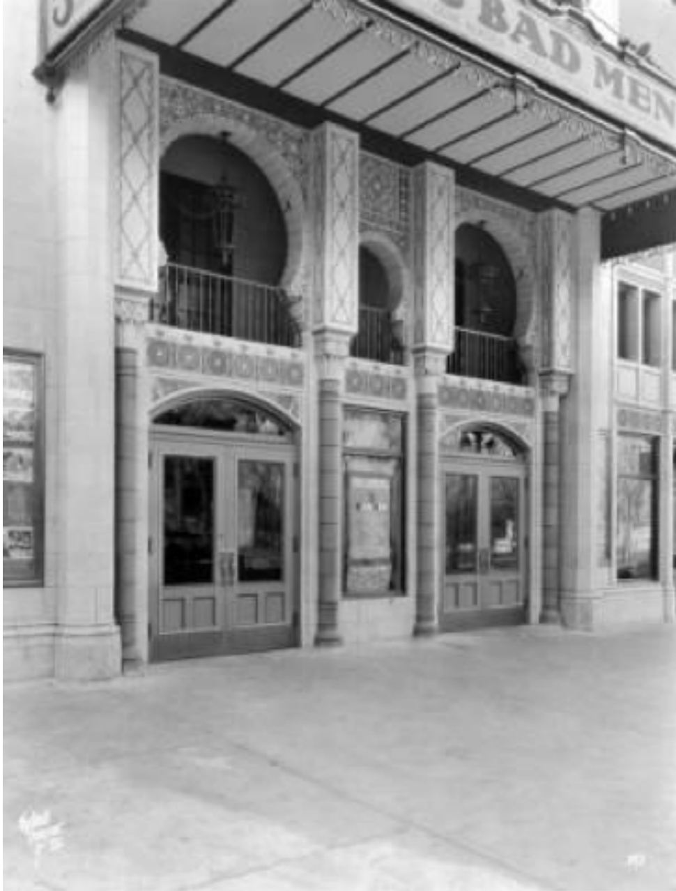
Figure 24. Detail of Aladdin Theater entrance revealing no exterior ticket window, but revealing elaborate unglazed terra cotta and elaborate polychrome (vivid contrasting colors), 1926. 126
