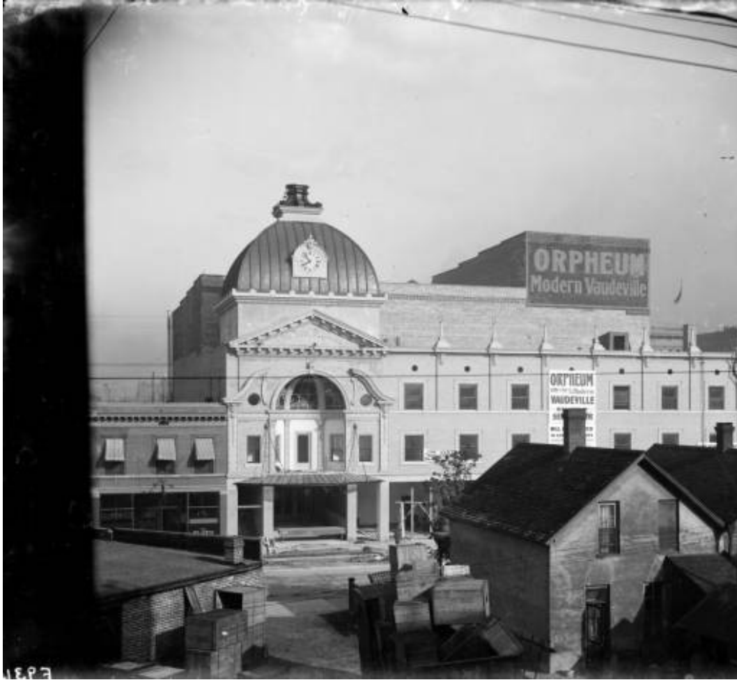
Figure 15. Denver's Orpheum Theater at 1517 Welton Street, c. 1910-1920. 62
