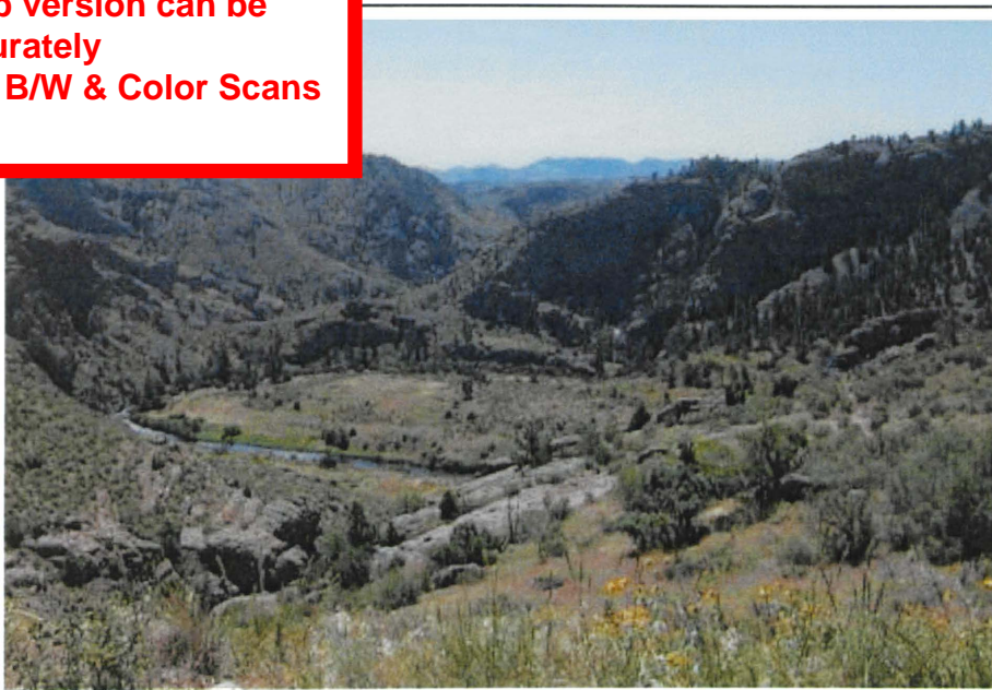
Figure 5 Phantom Canyon, looking south-southeast
