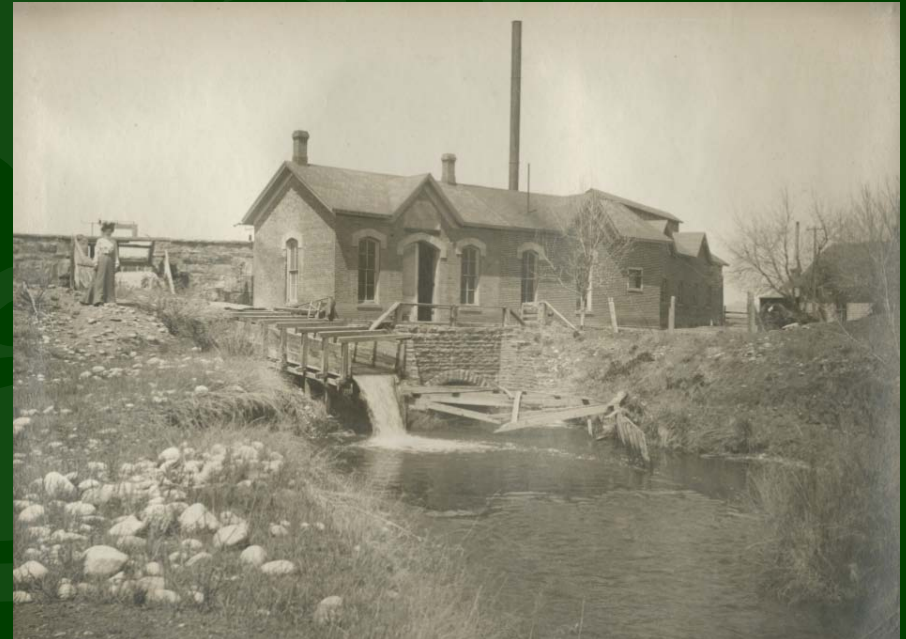
Fort Collins Water Works Pump House (1904)
