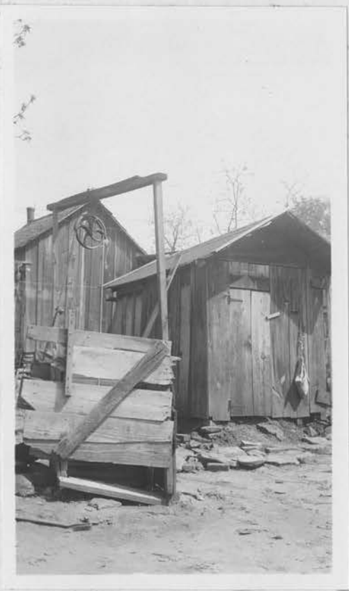
Fig. 6.--Open type unsanitary well.
