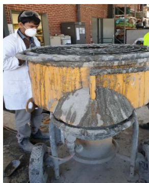
(a) Concrete mixing
