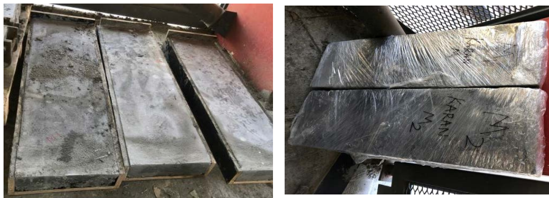
Fig. 5. Demolding of wall panels and curing with plastic wrap.
