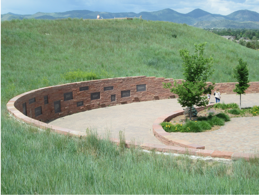
Figure 3. The Wall of Healing extends into the side of Clement Hill. Photo by Jena Schwake.
