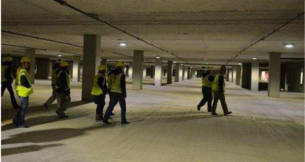
Figure 10: Folsom Parking Garage during construction, University of Colorado Boulder: Source, (CUBoulderToday, 2015)
