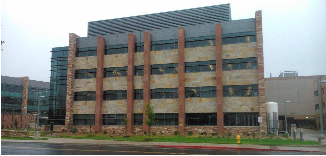
Figure 2: Chemistry Building: Source, Author
