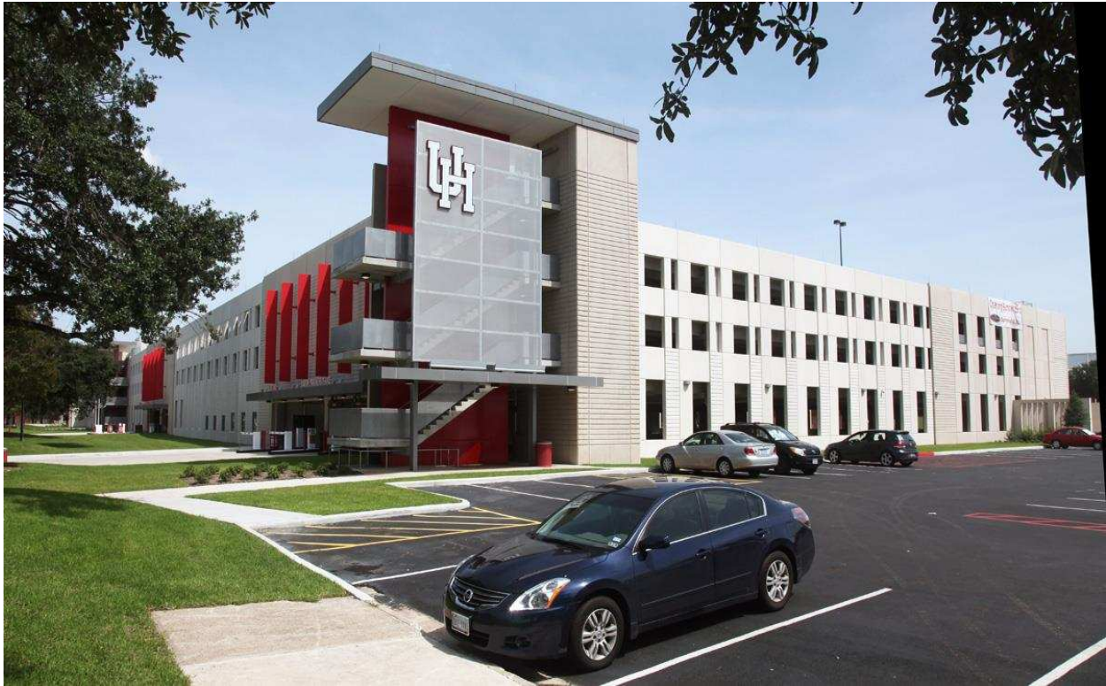
Figure 7: Stadium Parking Garage, University of Houston: Source, (WHRArchitects, 2012)
