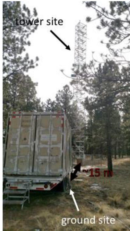
Figure A3.5. Photo of Manitou Experimental Forest Observatory (MEFO) shows the two separate locations where inlets were installed: the tower site and ground site. Sites were horizontally separated by ~15 m.
