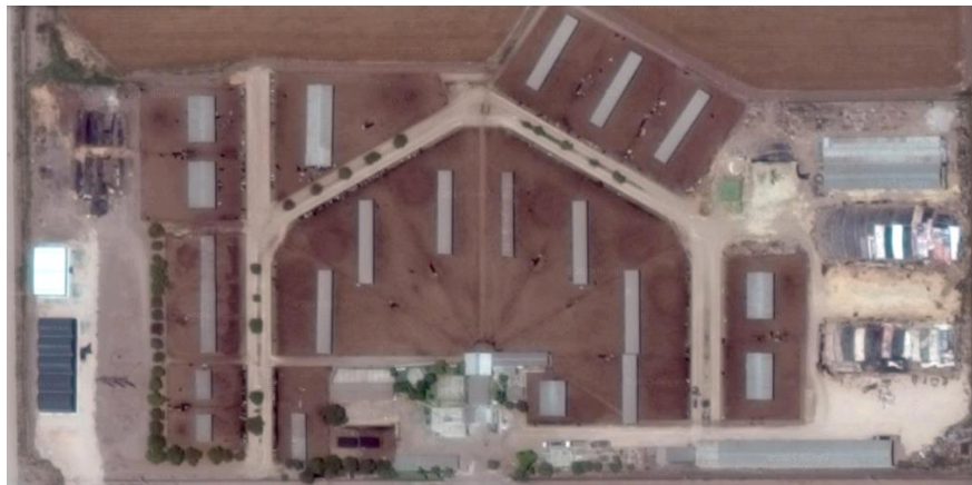
Figure 3.2. Aerial view of the housing structure of Farm1.
