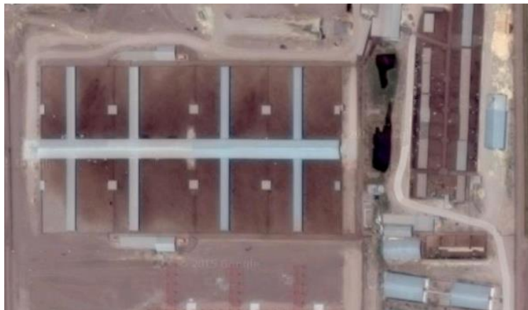
Figure 3.4. Aerial view of the housing structure of Farm 3.
