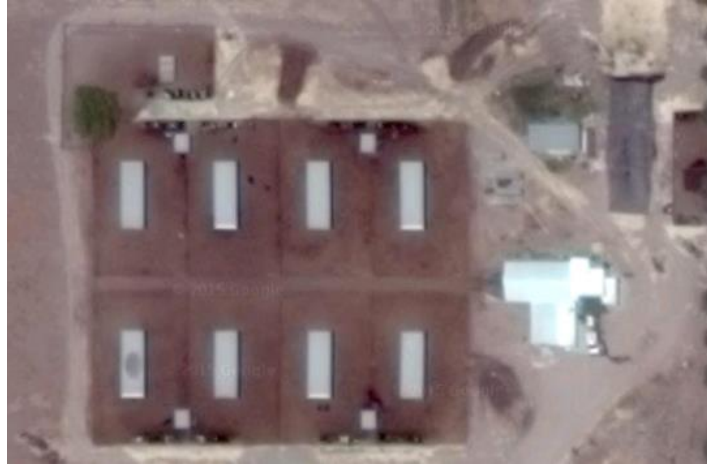
Figure 3.3. Aerial view of the housing structure of Farm 2.
