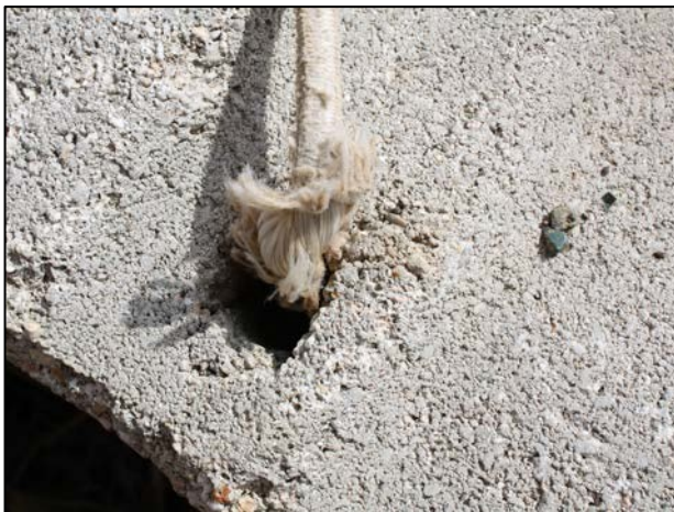
Figure 5. Photos Showing Damage to Bottom of ACB Armoring Following Overtopping of Portugués Cofferdam (Photos Courtesy of USACE)
