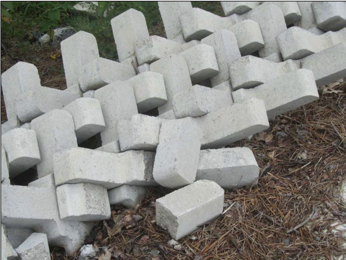
Figure 17. Photographs Showing Armoring Units Damaged from Vandalism
