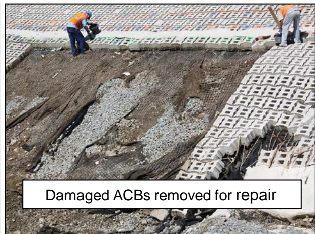
Figure 5. Photos Showing Damage to Bottom of ACB Armoring Following Overtopping of Portugués Cofferdam (Photos Courtesy of USACE)
