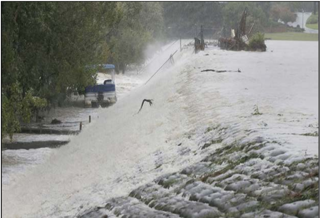
Figure 14. Photograph of Forest Lake Dam Showing Overtopping of Embankment Dam Armored Using Fabriform ACB System during Hurricane Joaquin
