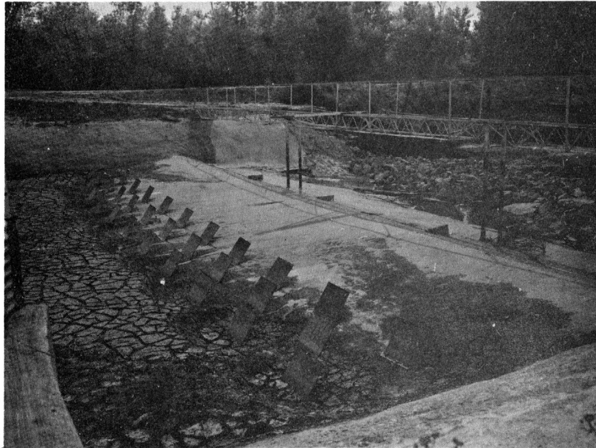
(b) Weir baffles, sill, and footbridge.
