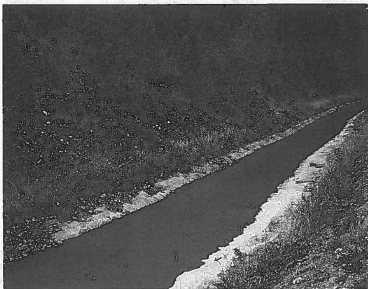
Fig. 2 Plastic lining of a rock/earth canal
