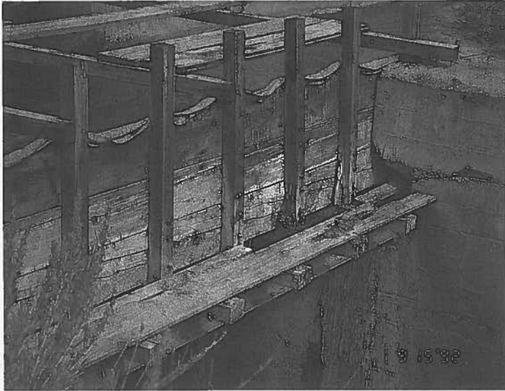
Fig. 4 A wood/concrete structure after repair
